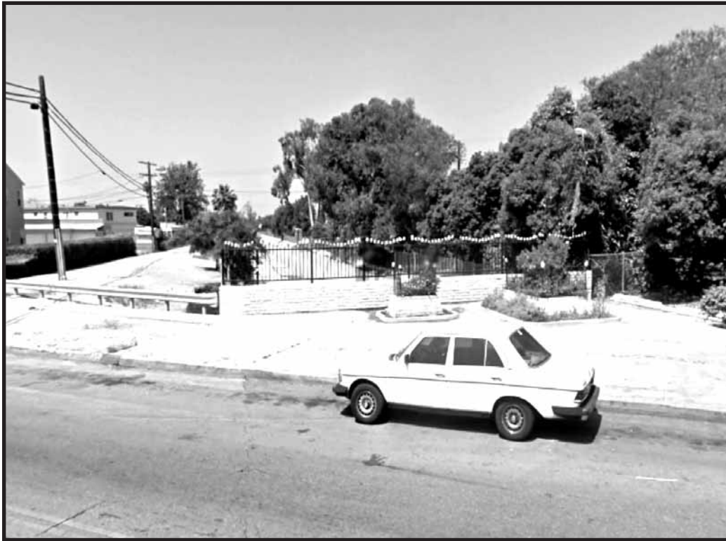
Ballona Creek. Looking west where Ballona Creek crosses under Hauser Street.
