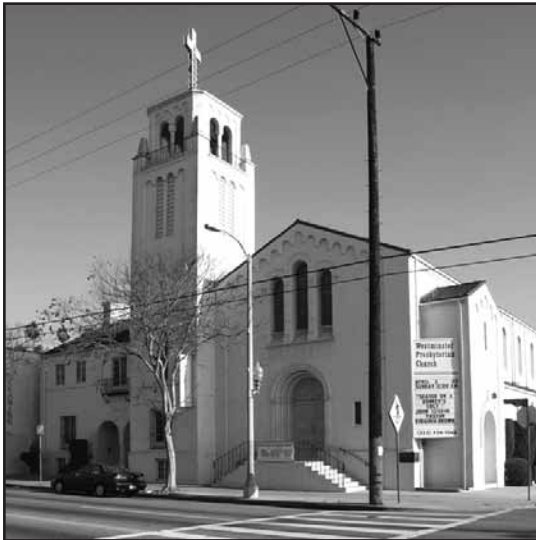
Westminster Presbyterian Church Building located at 2230 W. Jefferson Boulevard near 3rd Avenue.
