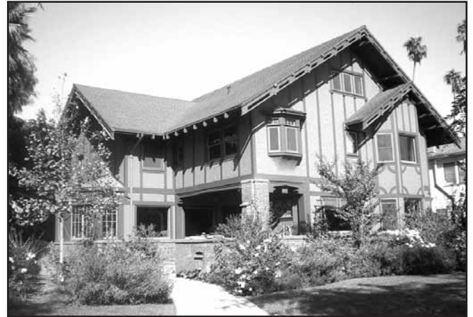
Holmes-Shannon House located at 4311 Victoria Park Drive.
