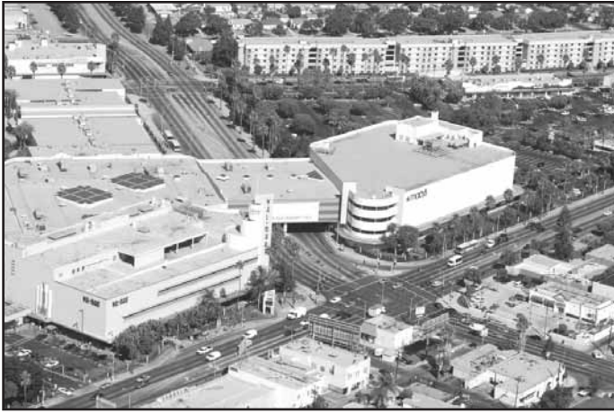
Former May Company Department Store (Now Baldwin Hills-Crenshaw Plaza) - Crenshaw/Martin Luther King Jr. Boulevards
