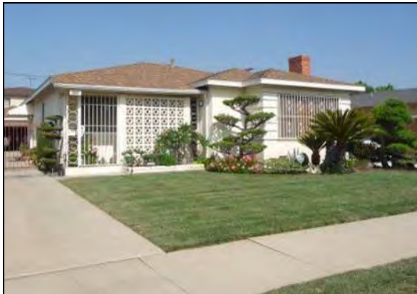
Address: 3811 S. Norton Avenue (contributor to the Crenshaw Seinan Historic District) Date: 1956
