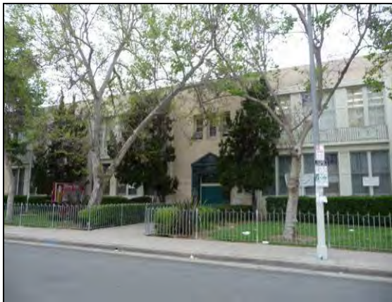
Address: 1700 S. Bronson Avenue Name: Arlington Heights Elementary School Date: 1936
