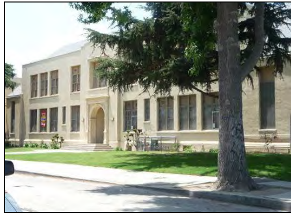
Address: 5939 S. 2 nd Avenue Name: 59 th Street Elementary School Date: 1928
