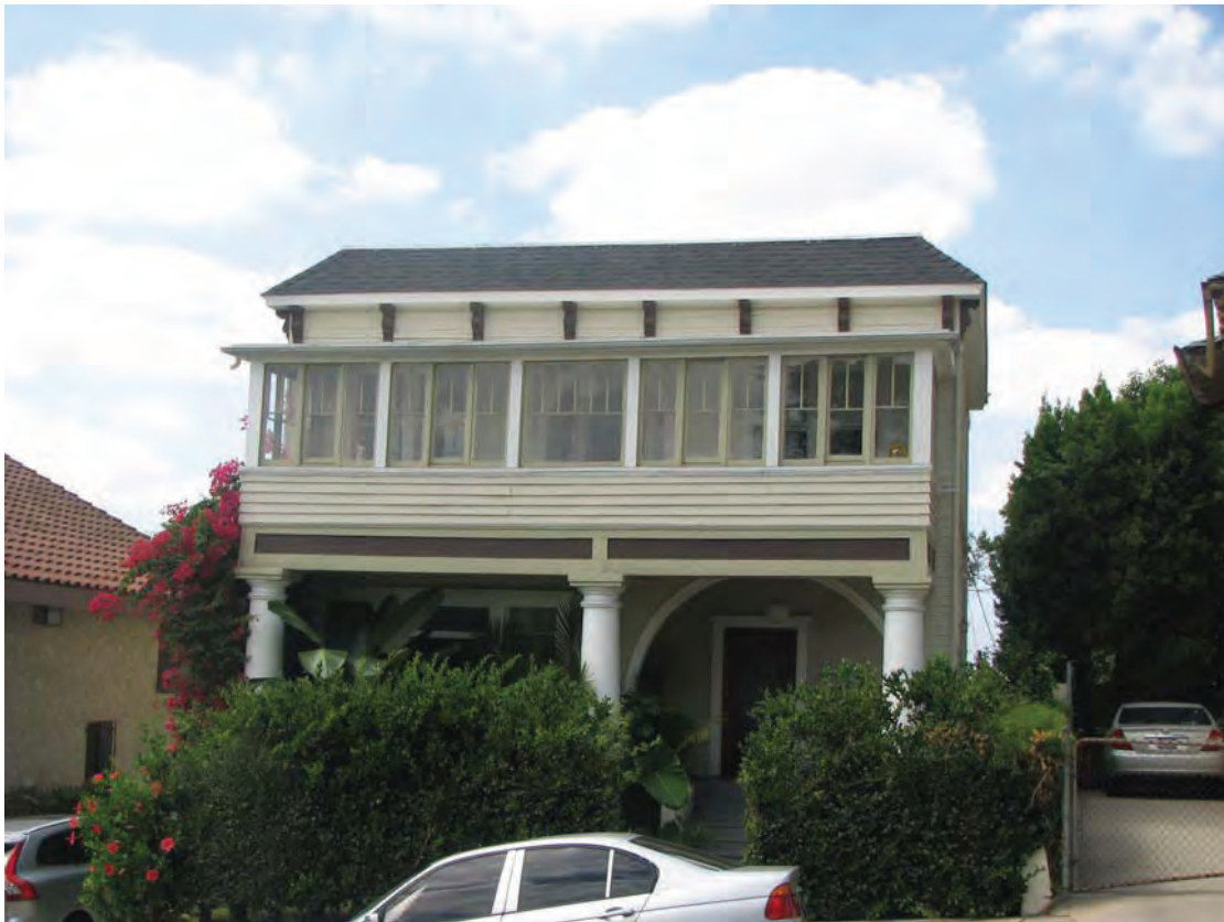
Restovich House, 1001 Everett Street, September 19, 2014 (Photograph by Charles J Fisher)
