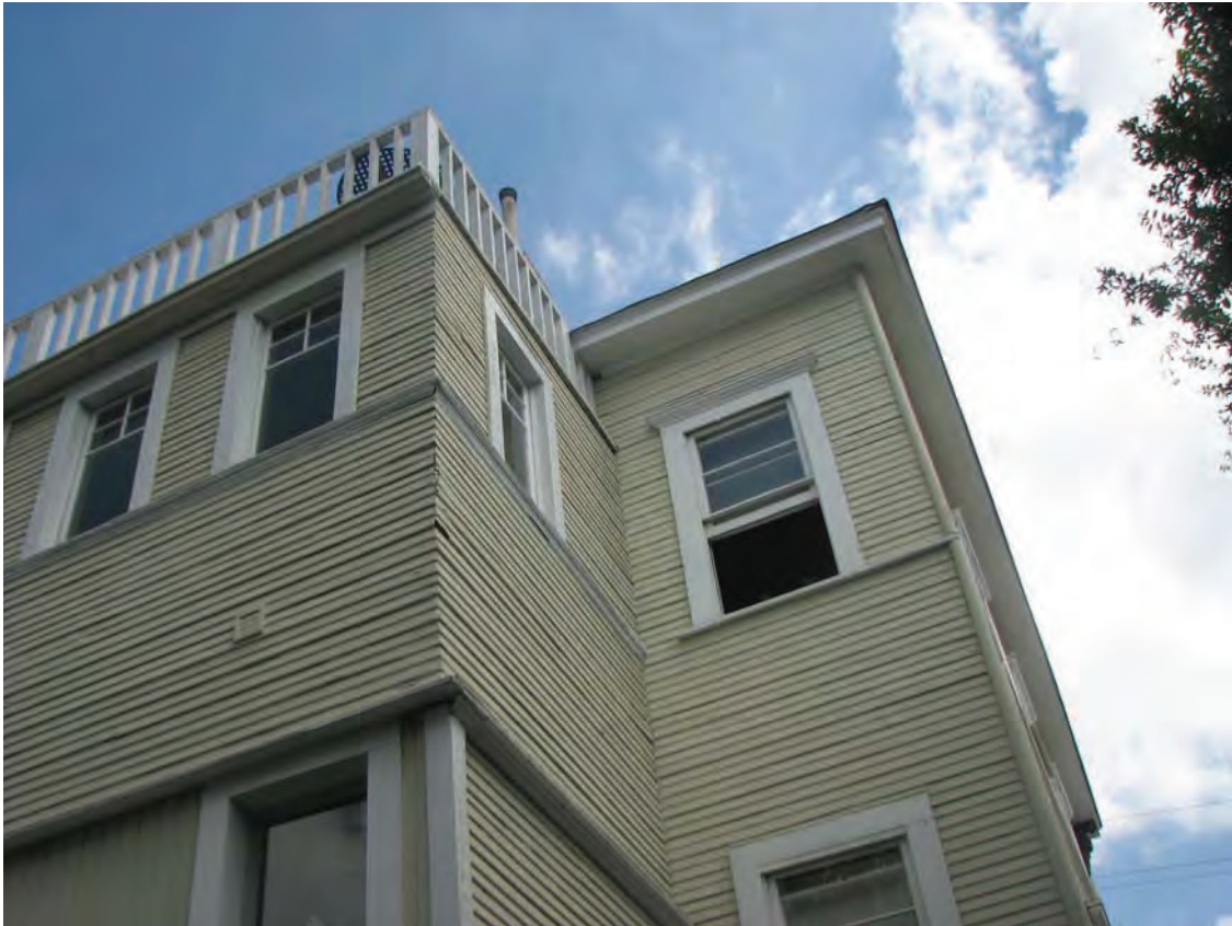
Restovich House, Southwest corner 1001 Everett Street, September 19, 2014 (Photograph by Charles J Fisher)
