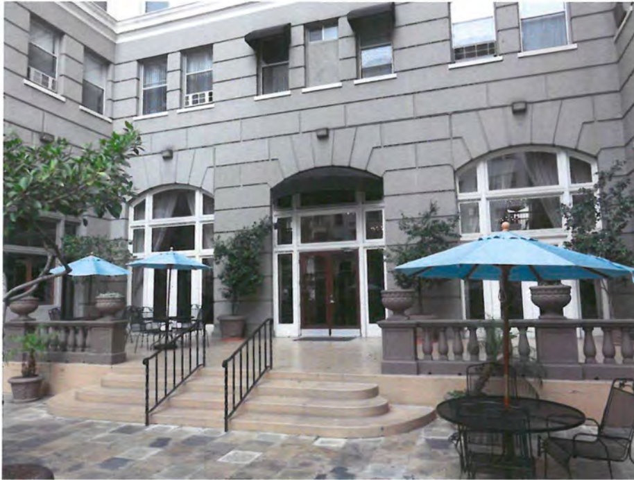
Original entrance on west elevation at apex of U-shape.
