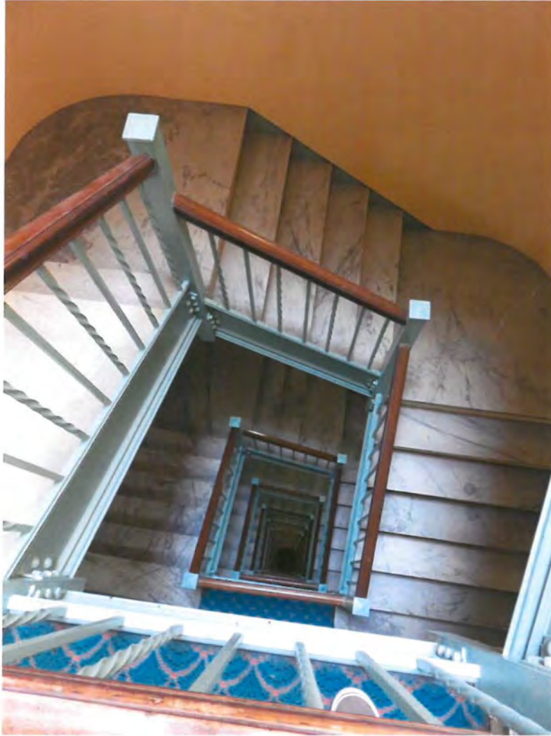
Primary internal staircase. Note marble treads and iron balusters supporting wood handrail.
