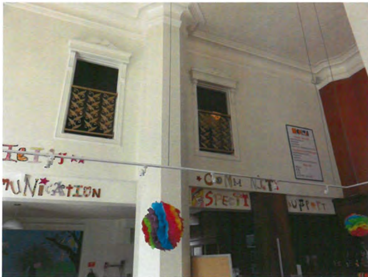
2 nd floor in corner retail unit
