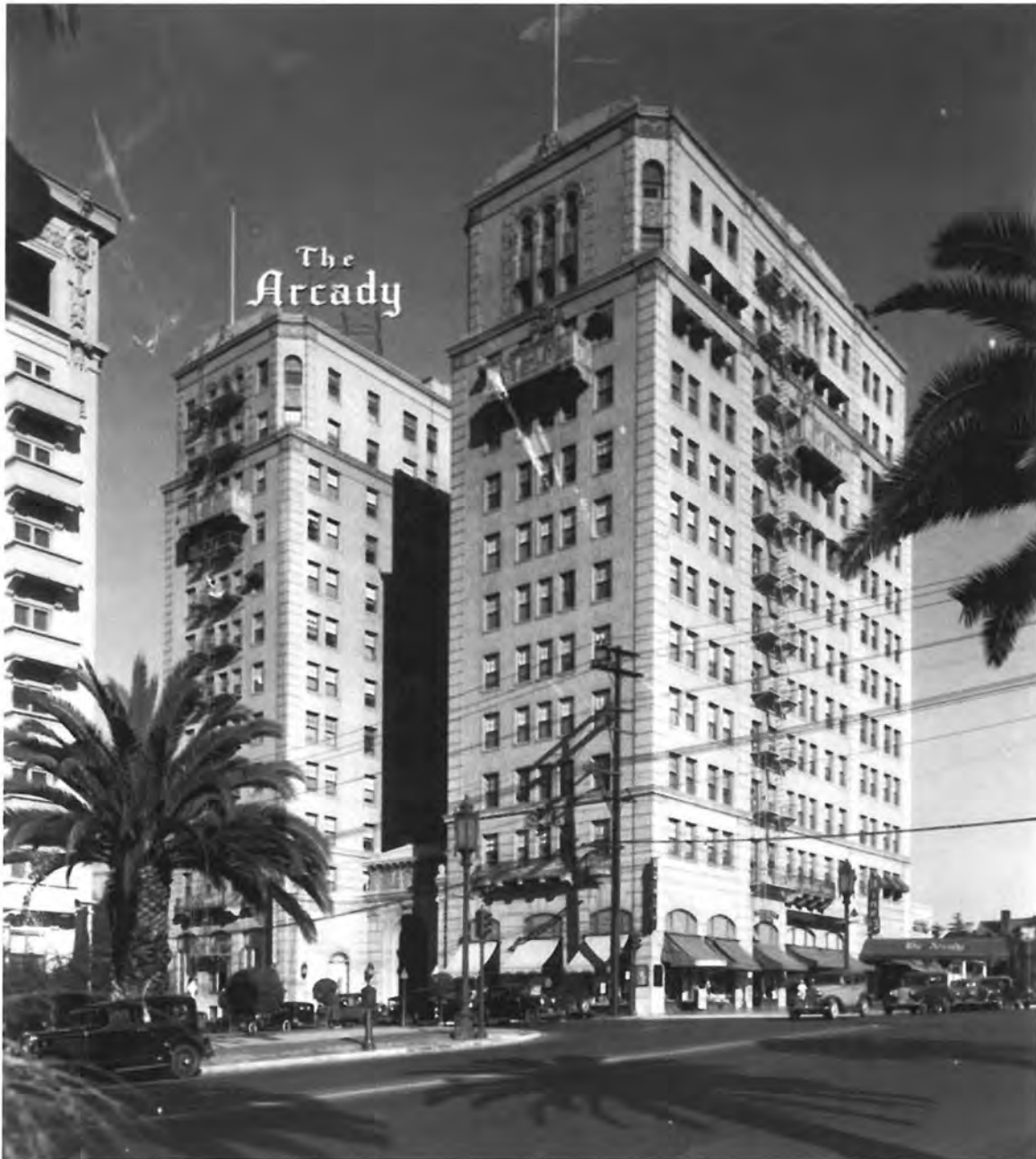
Historic image, circa 1927, showing west elevation with original entrance on Rampart Boulevard, and south elevation along Wilshire Boulevard.
