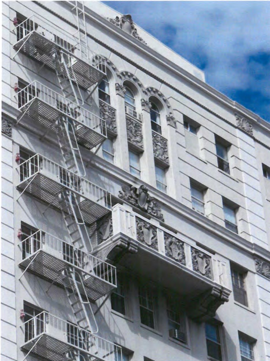
Cast stone detailing, upper stories, and south elevation.
