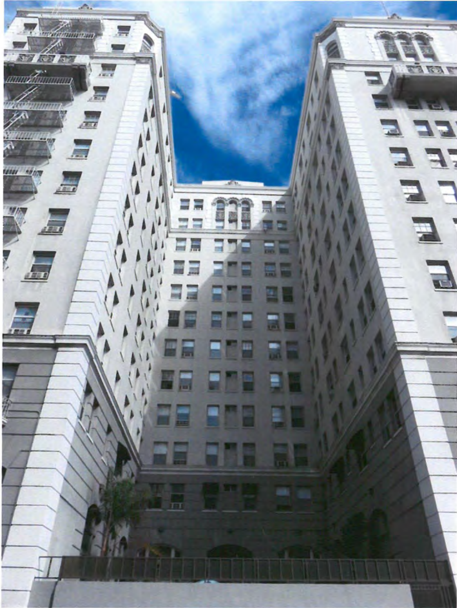
View illustrating U-shaped form, and internal wall of west elevation.
