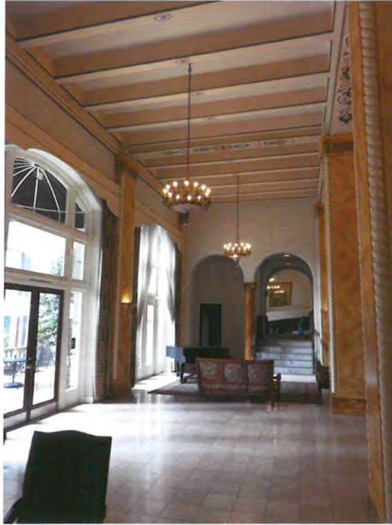
Foyer and lobby area, looking west Note ornamental column and stair balustrade. Note pilasters, capitals, and rope moldings that is original. Floor tile is replacement ceramic material.
