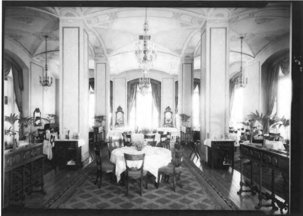
Historic Image, ca. 1927, interior of Dining Room
