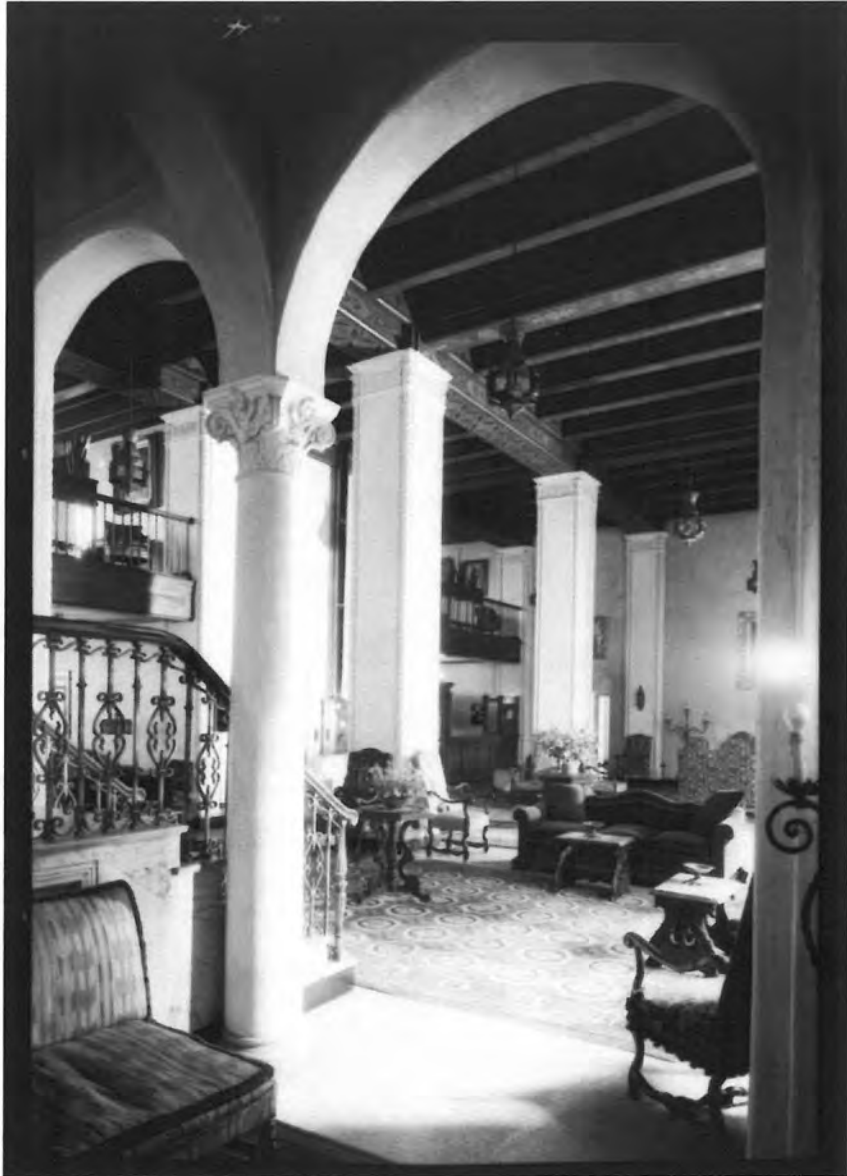
Historic Image, circa 1927, main lobby, showing original materials, paint scheme and furnishings
