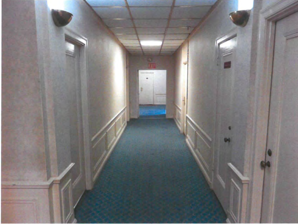
Internal corridor, upper stories, illustrating typical millwork and wainscoting.
