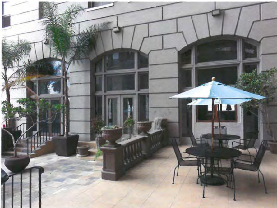
Original entrances and arched openings flanking internal courtyard.
