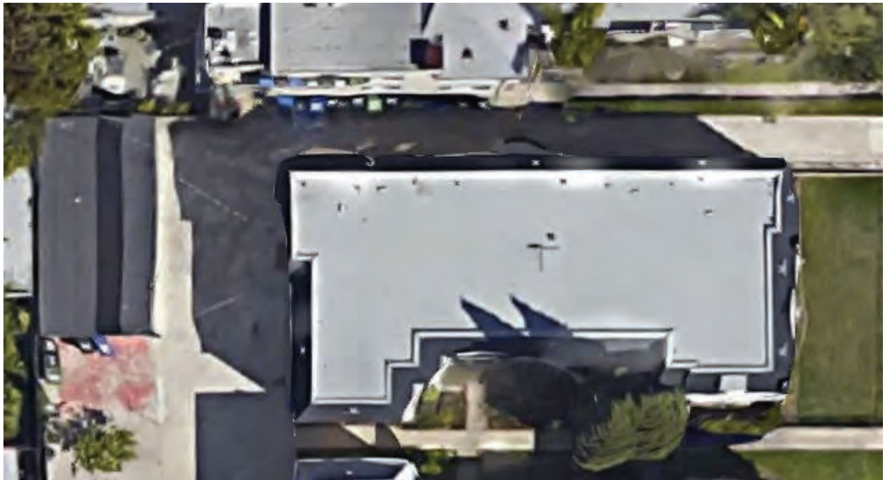
Spinning Wheel Apartments, satellite view, 423-27½ N. Hayworth Avenue, c 2015 (photograph by Google Earth)
