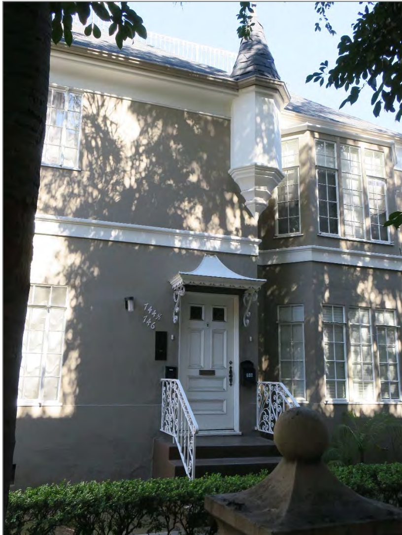
Courtyard unit entry and turret on south façade, view to northeast (ARG, 2017).
