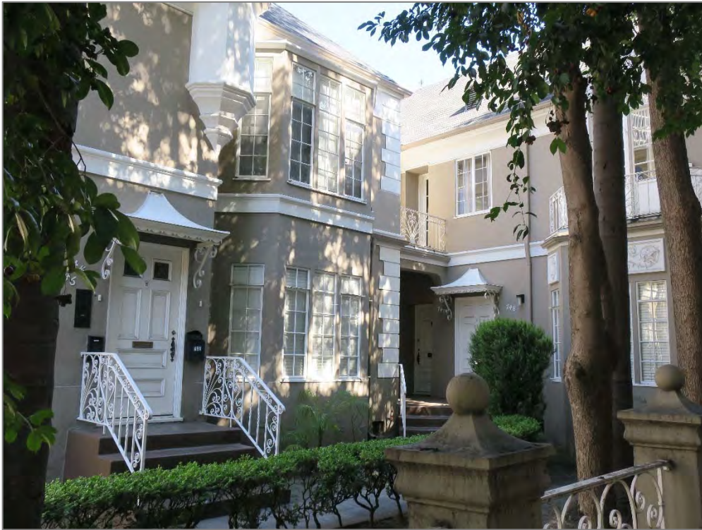
South and west courtyard façades with corner stoop, view to northeast (ARG, 2017).
