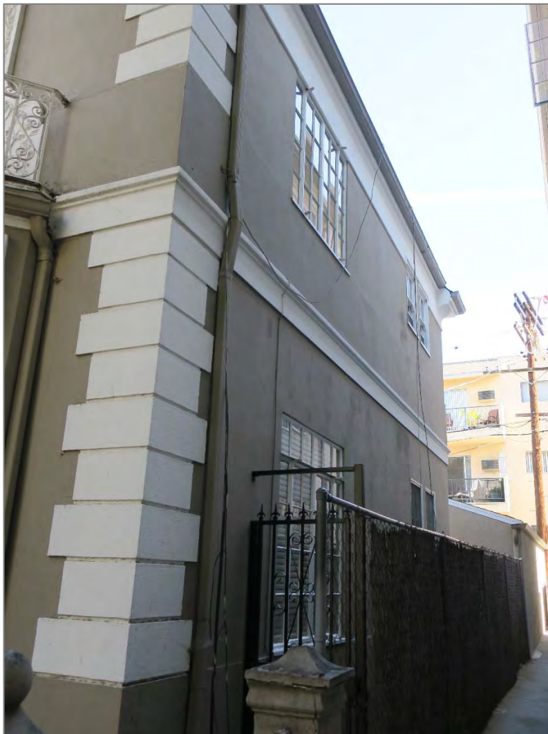
South façade, view to northeast (ARG, 2017)
