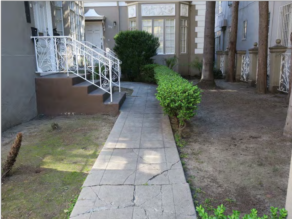
Courtyard and walkway, view to east (ARG, 2017).
