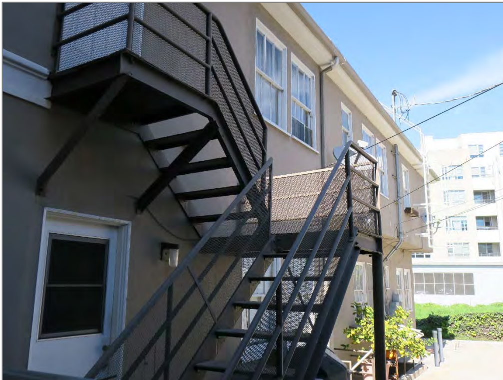
East façade, view northwest (ARG, 2017).
