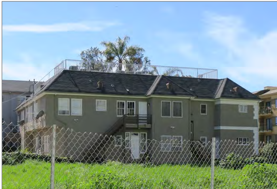
North and east façades, view southwest (ARG, 2017).
