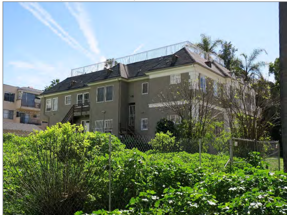
North and west façades, view southeast (ARG, 2017).
