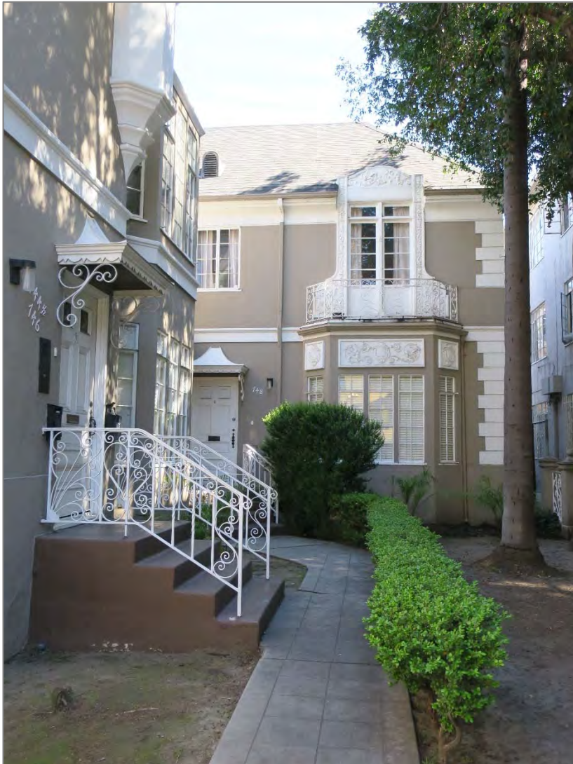
Courtyard unit entries, view to east (ARG, 2017).
