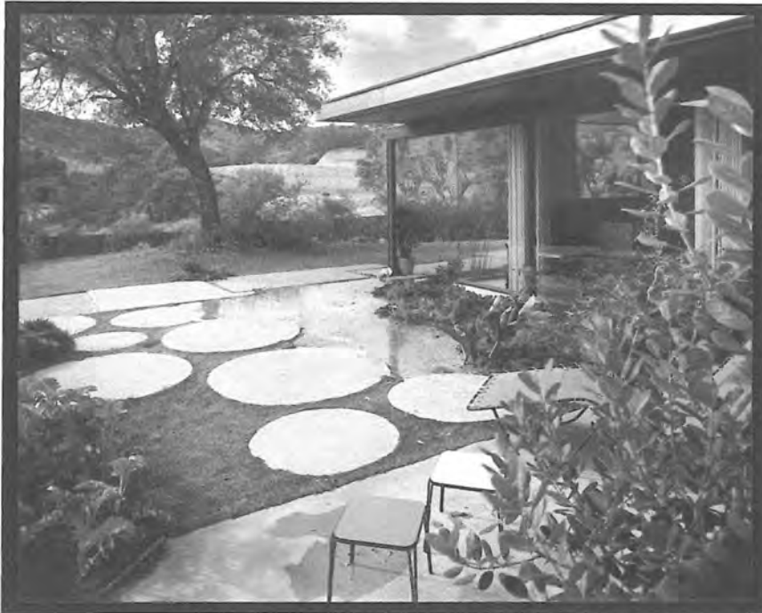
Historic Figure 3. Rear Façade, SE corner of building. Milton Goldman House, 1953. Photo by Julius Shulman. Camera facing SW. © J. Paul Getty Trust. Getty Research Institute, Los Angeles (2004.R.10)
