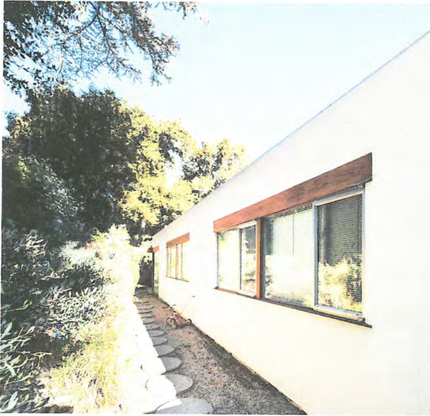
Contemporary Figure 7. North elevation. Camera facing E. Milton Goldman House, 2016. Photo by Darren Bradley.
