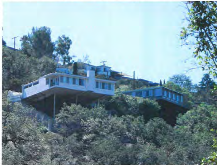
Neutra-designed stilt houses in the Platform House Historic District
