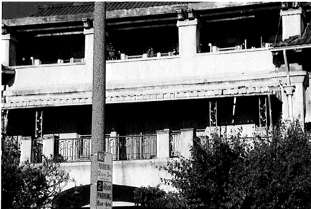
Third floor: Original roof tiles, pergola, brackets and piers remain, as do windows. Second floor: Added awning and supports and some window changeouts. Original half-height piers with original metal trim, original copper gutters, now painted, view west.
