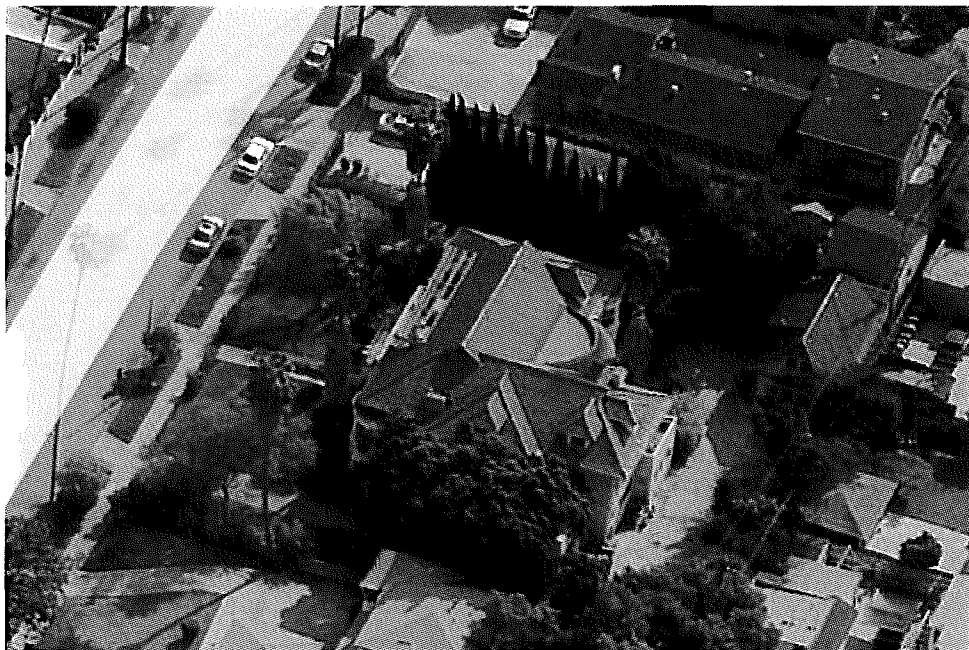
Residence and garage: View southeast. Source: Bing Maps.
