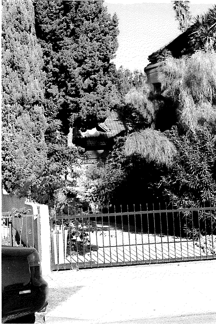
Slight view, garage at southwest of residence, behind greenery.
