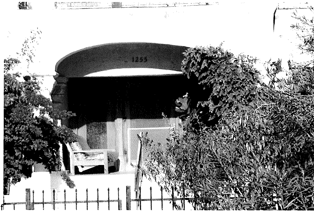
Entry: Pillars with capitals at rear. Glass in entry door and sidelights has been changed out. View west.
