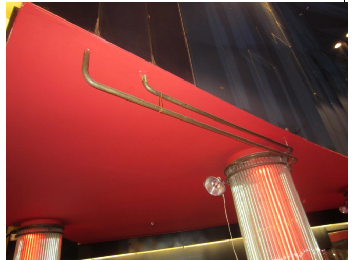
Brass Decorative Ceiling Features near Column just east of stairway, 2014
