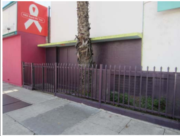
North Elevation, View Southeast
