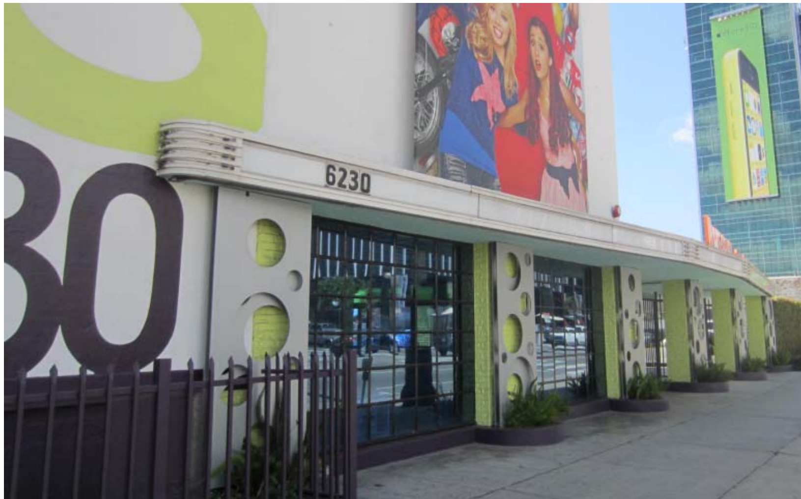
Detail of western end of north elevation, showing fenestration, piers, and semicircular planters, view southwest (PCR 2014)
