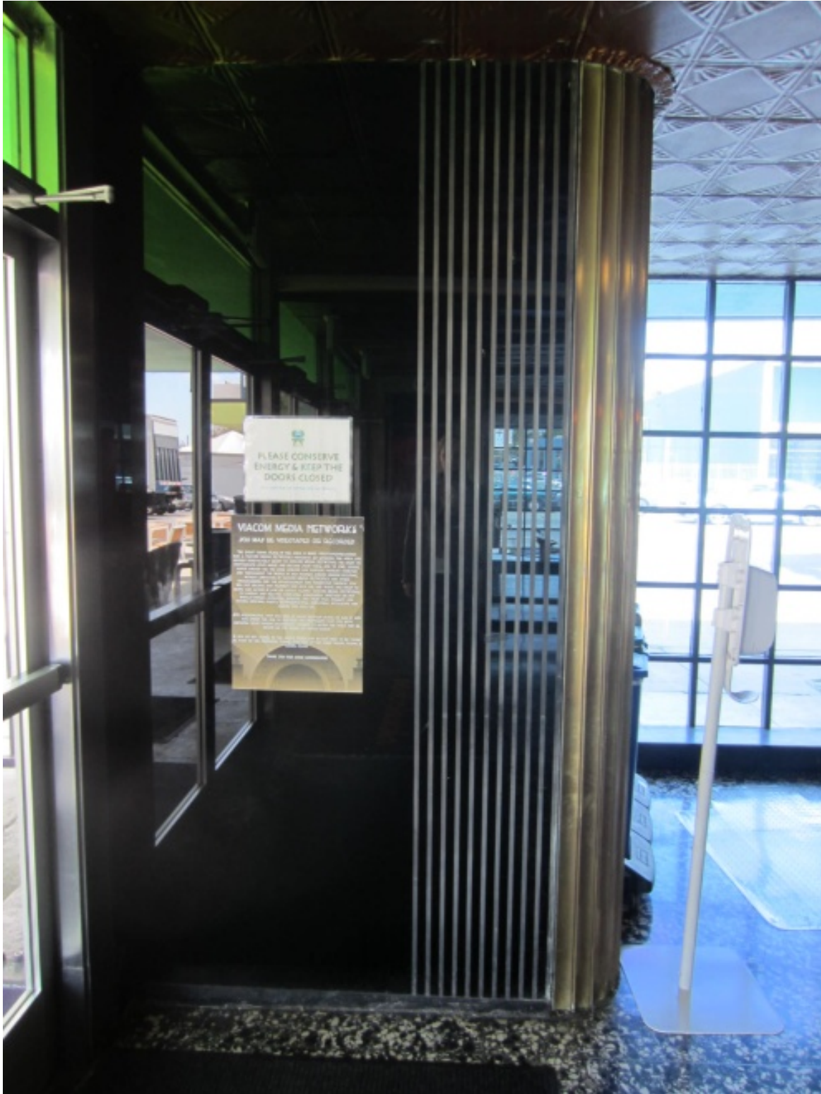
Black structural glass wall and attached fluted column north of entrance (PCR 2014)
