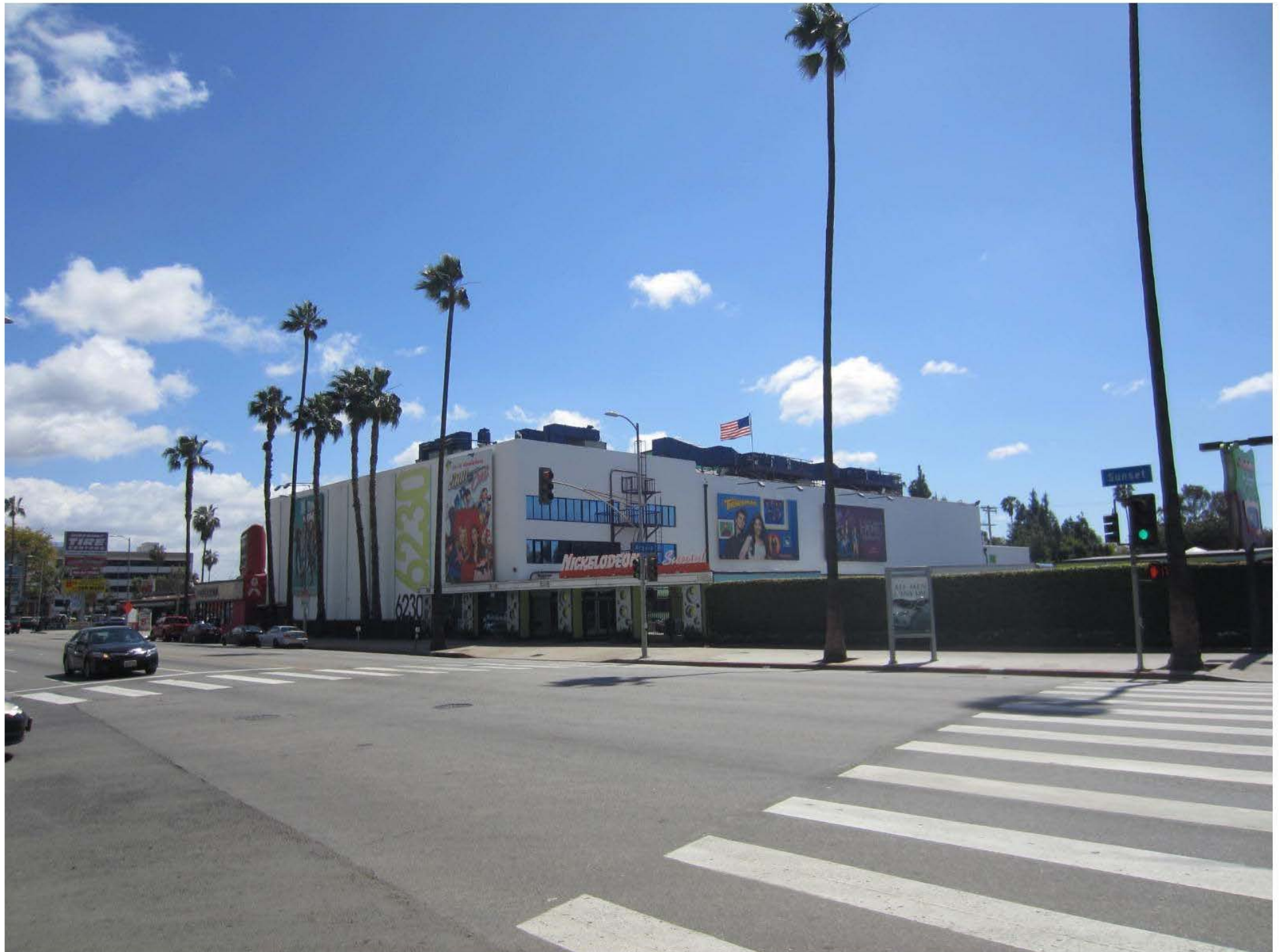
Earl Carroll Theater Building, 6230 Sunset Boulevard, north and west elevations, view southeast (PCR2015)
