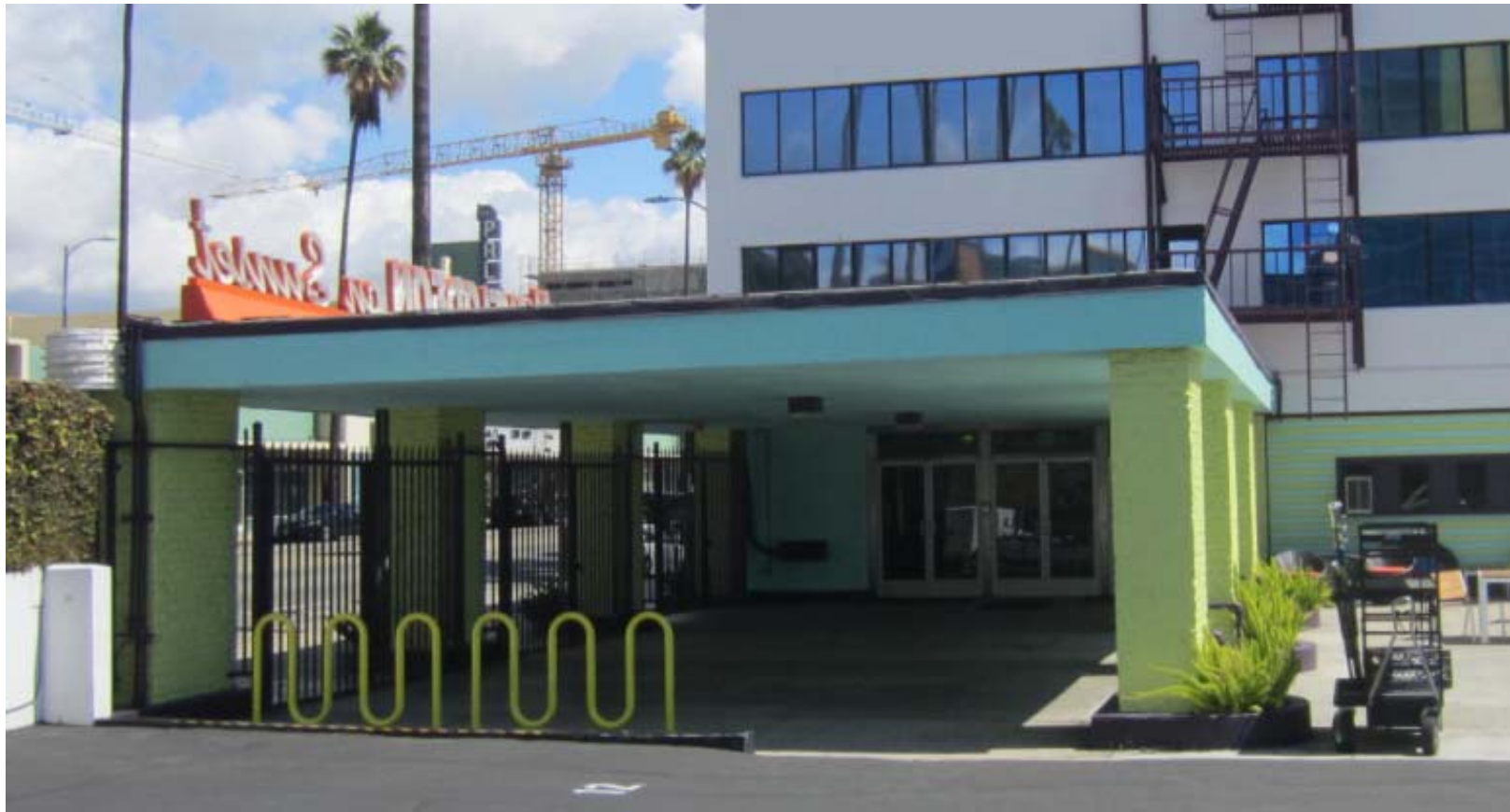
Porte-cochère and main entry, view east (PCR 2014)
