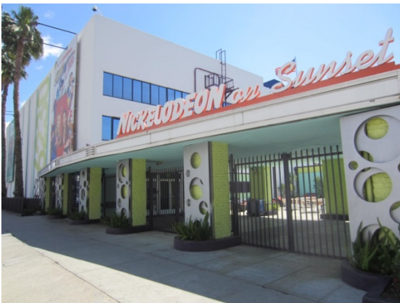
West Elevation, View Southeast
