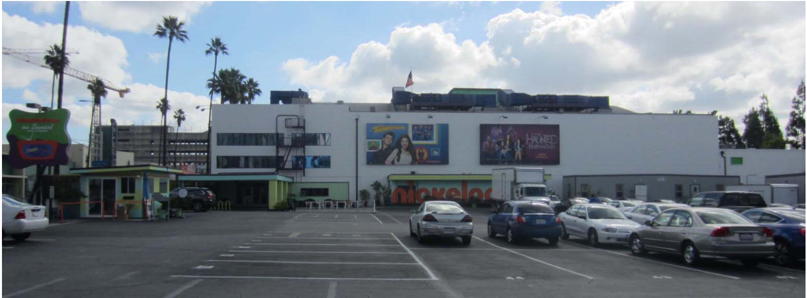
West elevation and parking lot, view east (PCR 2014)
