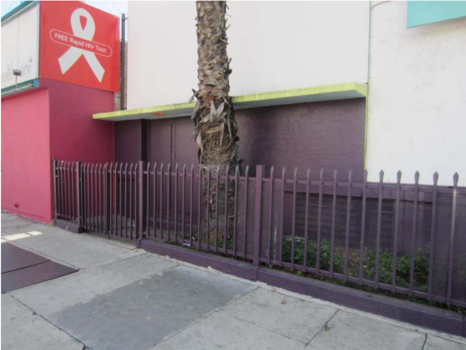
North elevation, view southeast (PCR 2014)
