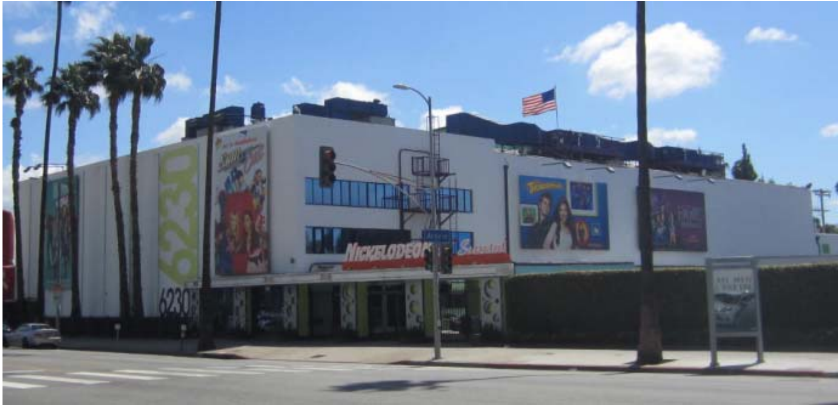
North and west elevations, view southeast (PCR 2014)
