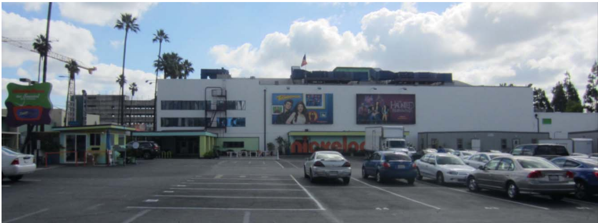
West Elevation, View East
