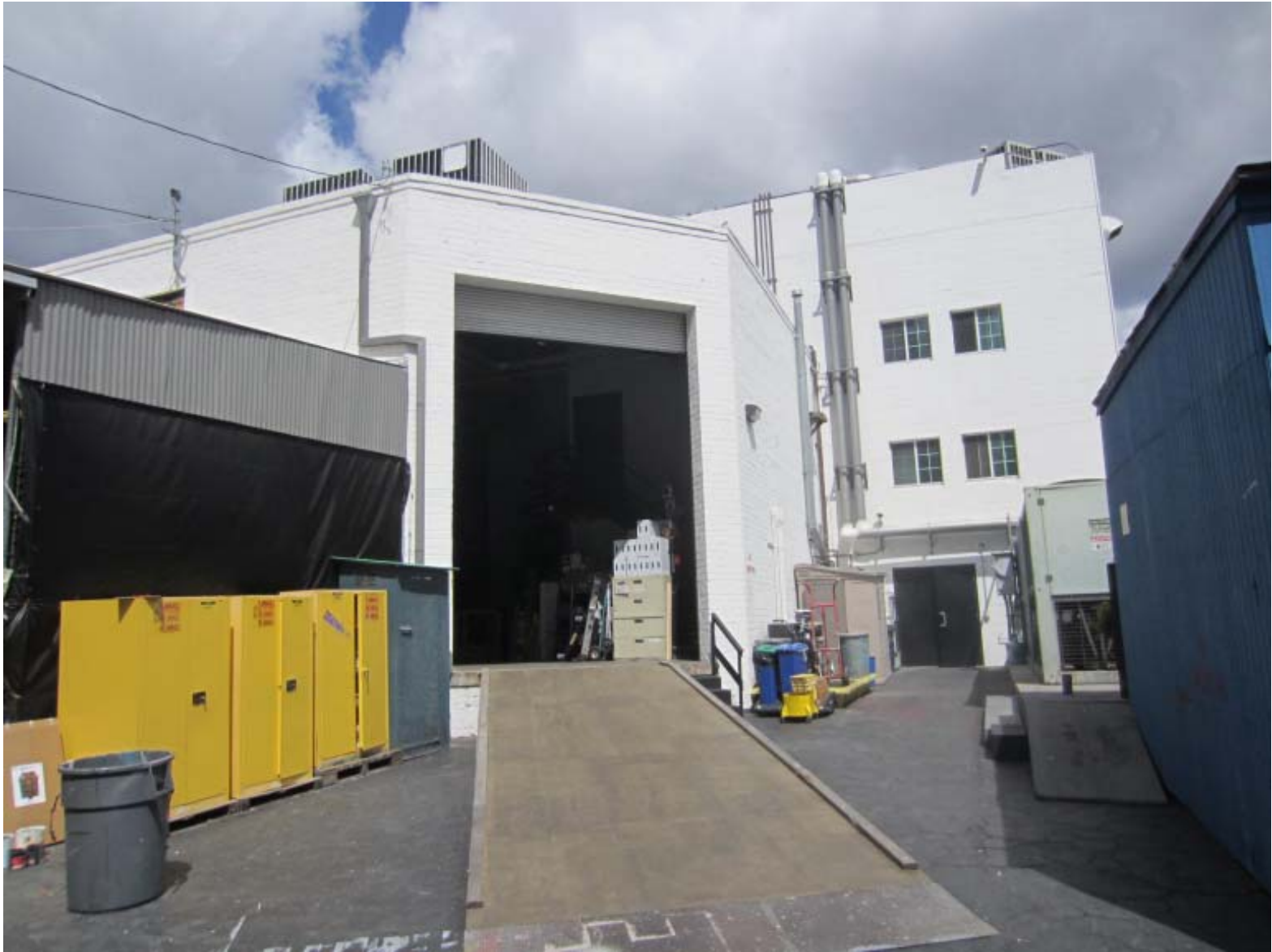
Addition to the rear (south) elevation, view north (PCR 2014)
