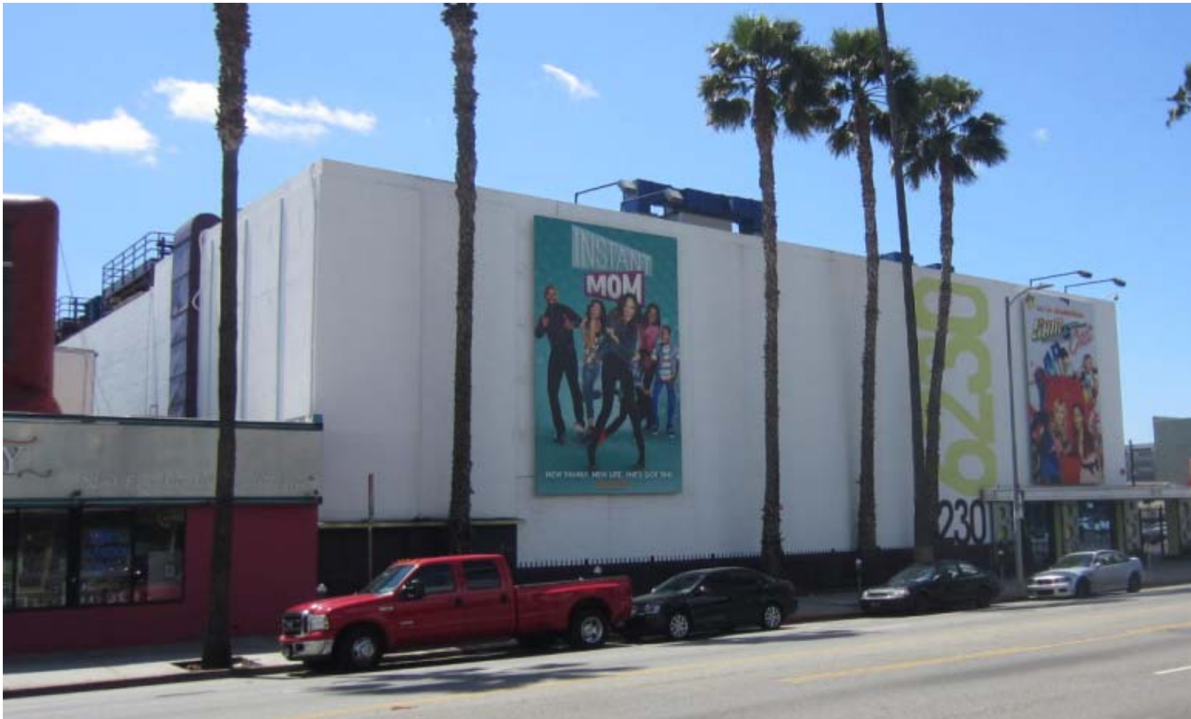
North and east elevations, view southwest (PCR 2014)
