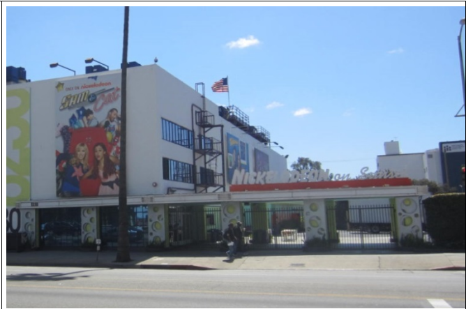
Porte-cochère, View South
