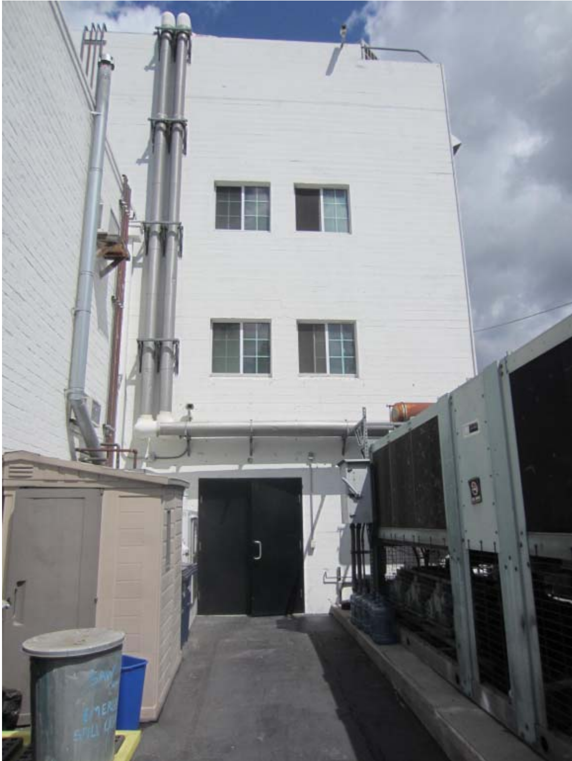
Original wall of rear (south) elevation, with original fenestration pattern, view north (PCR 2014)
