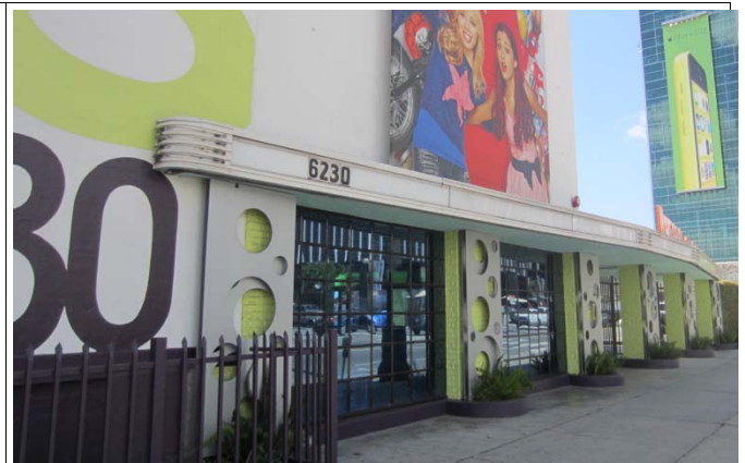
North Elevation, View Southwest
