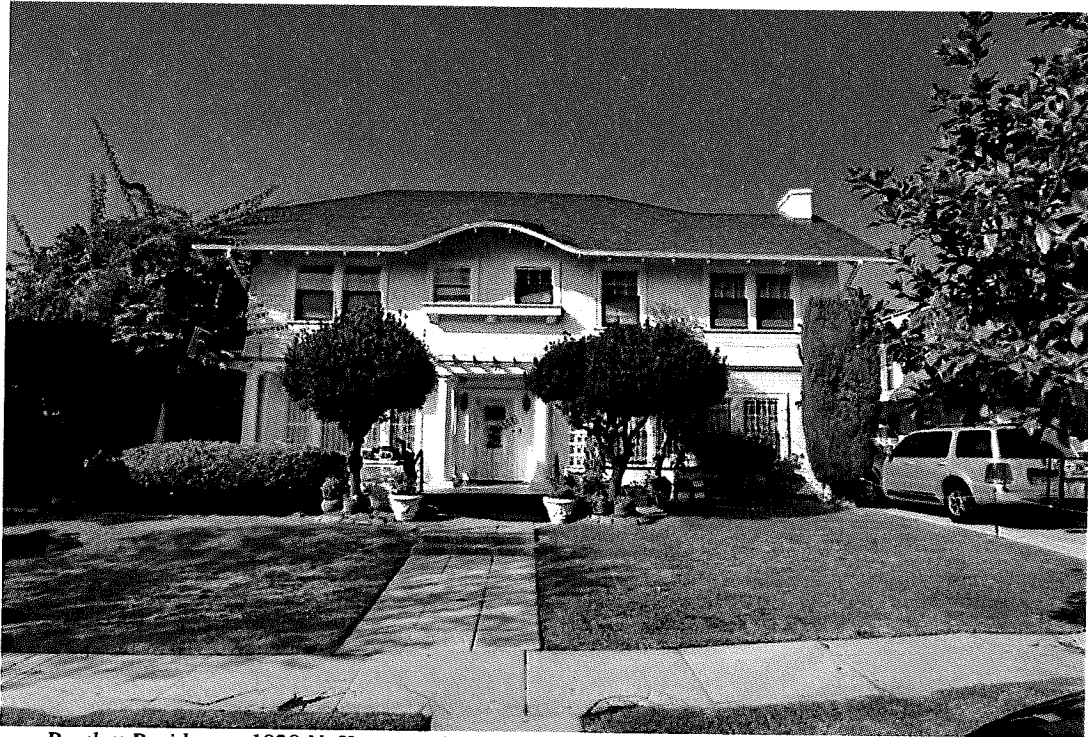
Bartlett Residence, 1829 N. Kenmore Avenue, October 31, 2011 (Photograph by Michael Locke)
