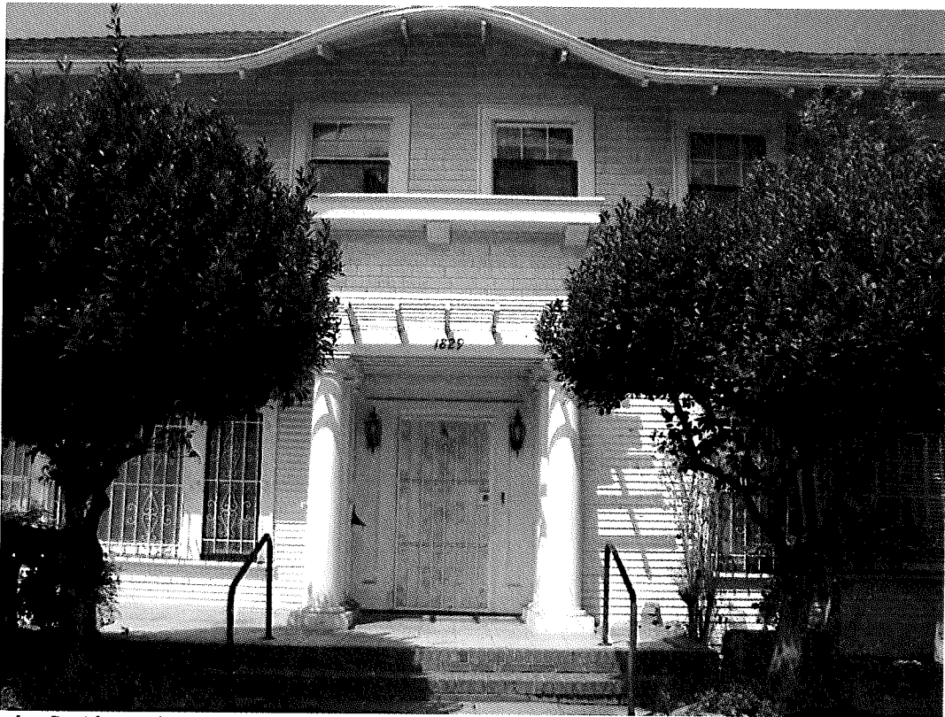
Bartlett Residence, front porch, 1829 N. Kenmore Avenue, August 7, 2014 (Photograph by Charles J. Fisher)
