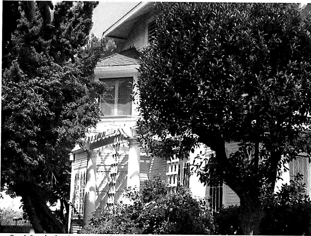
Bartlett Residence, South facade showing two story bay, 1829 N. Kenmore Avenue, August 7, 2014 (Photograph by Charles J. Fisher)
