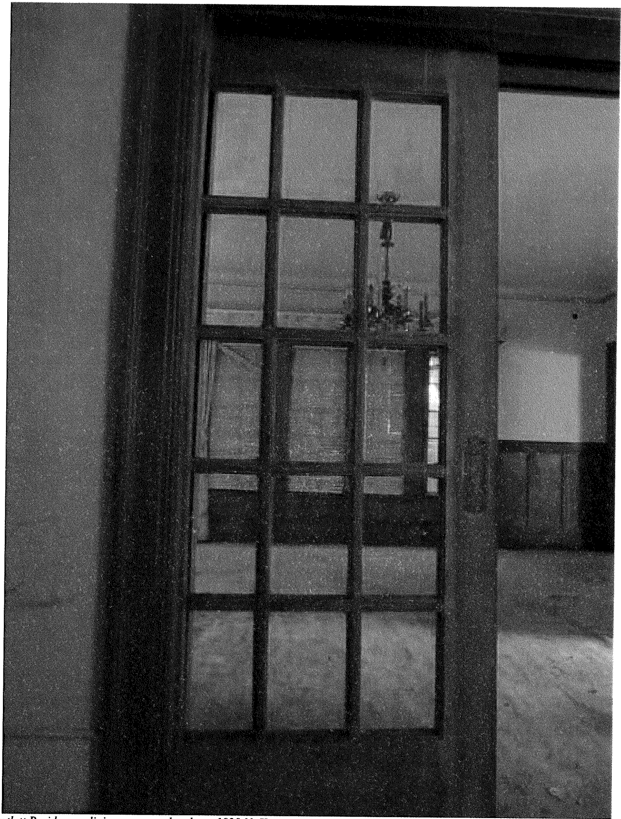
Bartlett Residence, dining room pocket door, 1829 N. Kenmore Avenue, January 2013 (Photograph by Abraham Soghomonian)
