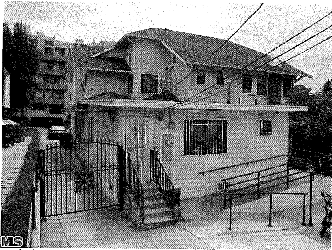
Bartlett Residence, rear facade, 1829 N. Kenmore Avenue, January, 2013 (MLS Photograph)
