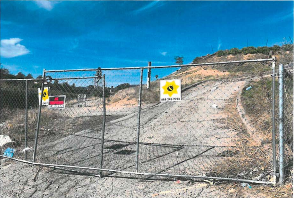
Photograph of entrance to the property off of Kagel Canyon Street
