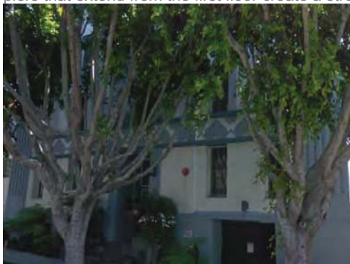
Art Deco Apartment Building, c. 1931
