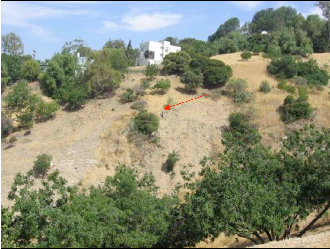
Fig. 19. Worker clearing a near-vertical slope using hand tools at Moss site (red arrow), apparently well outside the required 200' buffer from the house upslope. This particular worker cleared a large percentage of the remaining coastal sage scrub community at Moss during my brief visit (July 2008).
