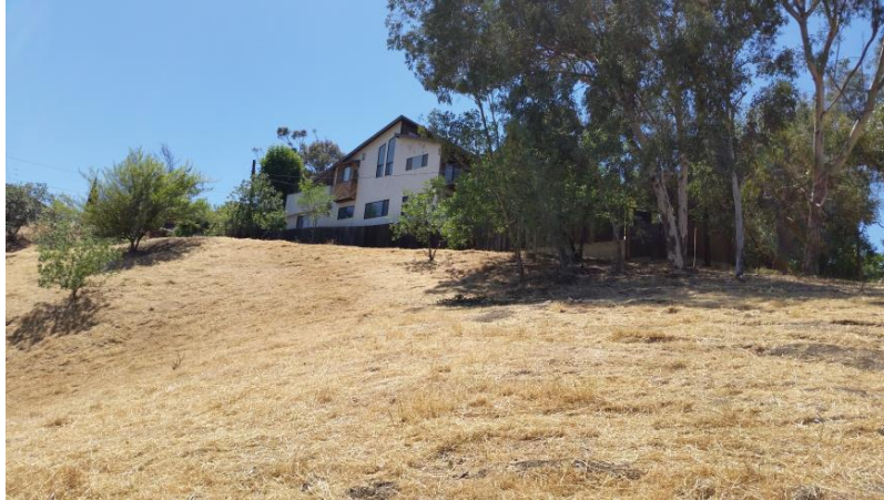
View of 3957 Brilliant Drive from the project site
