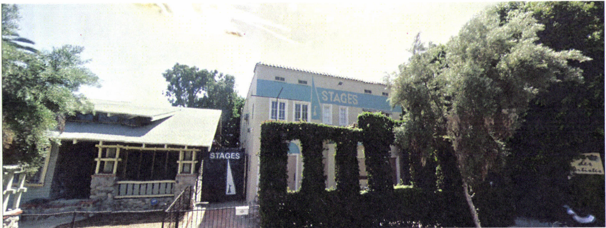
Photograph 17: View of Eastern side of McCadden Place
