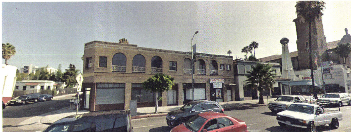
Photograph 2: View of Northeast corner of Sunset Boulevard and Las Palmas Avenue
