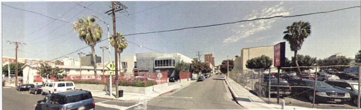
Photograph 27: View of North side of Selma Avenue at McCadden Place
