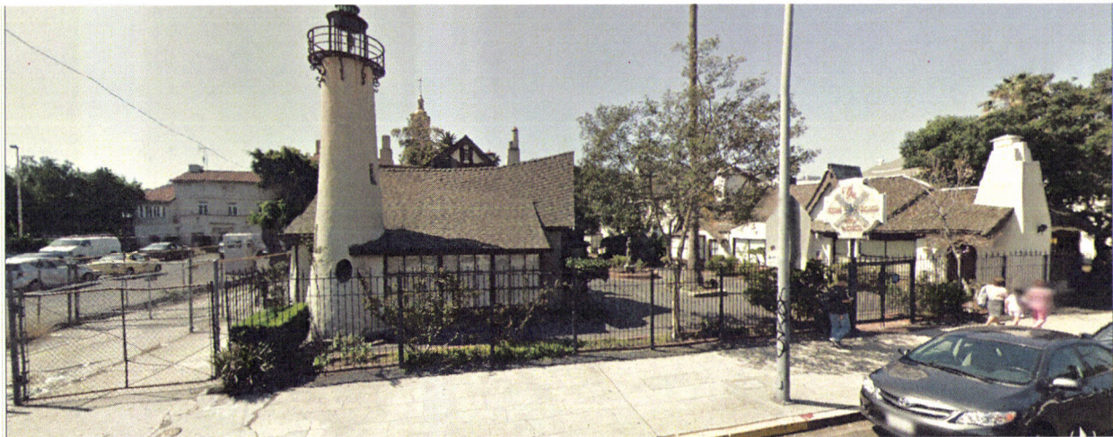
Photograph 5: View of existing Crossroads of the World from Selma Avenue
