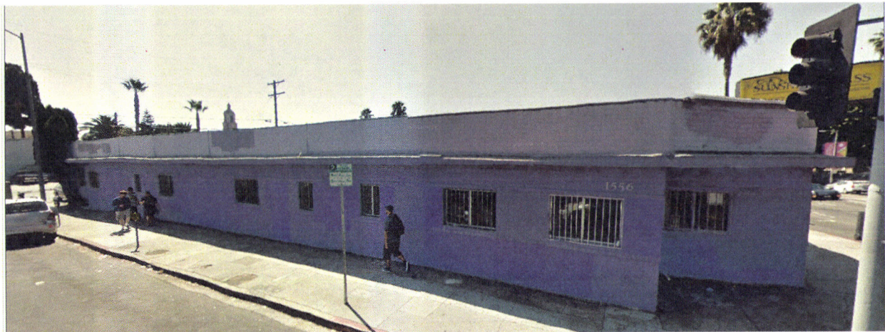
Photograph 14: View of Southeast corner of Selma Avenue and Highland Avenue
