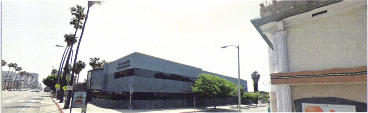
Photograph 22: View of Southeast corner of Sunset Boulevard and Las Palmas Avenue
