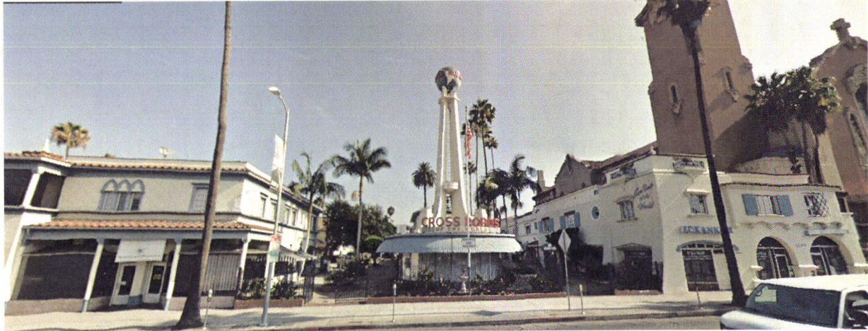
Photograph 1: View of Existing Crossroads of the World from Sunset Boulevard
