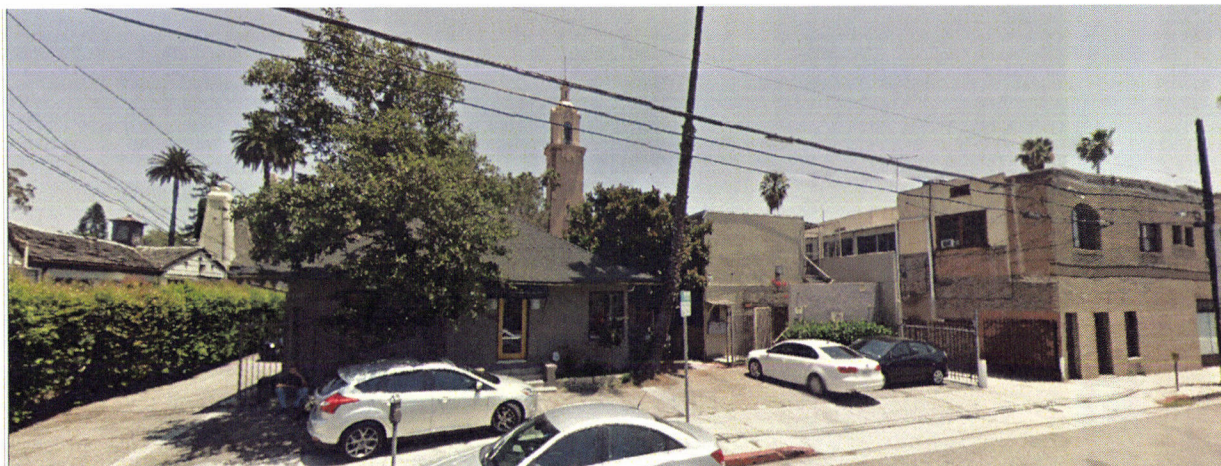
Photograph 3: View of Eastern side of Las Palmas Avenue
