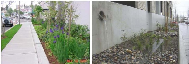
Infiltration planters allow water to infiltrate through the planter soil matrix and into the ground. Flow-through planters include the use of a waterproof lining and underdrain. Both types of planter boxes require an overflow to an approved stormwater conveyance system and may be used to help fulfill site landscaping requirements.
