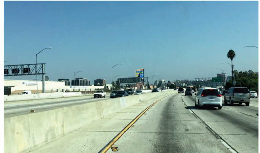
Photo F.720: I-110 Northbound view at 720 feet from 12th Place Sign
