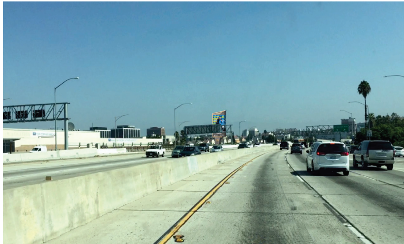
Photo G.290: I-110 Northbound view at 290 feet from 12th Place Sign
