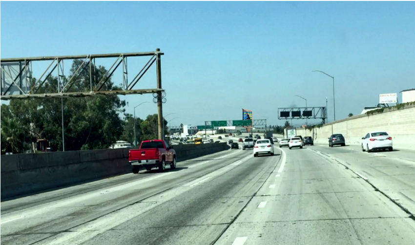
Photo B.1250: I-110 Southbound view at 1,250 feet from 12th Place Sign
