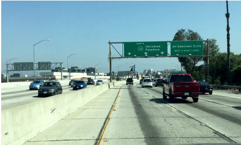
Photo E.1200: I-110 Northbound view at 1,200 feet from 12th Place Sign
