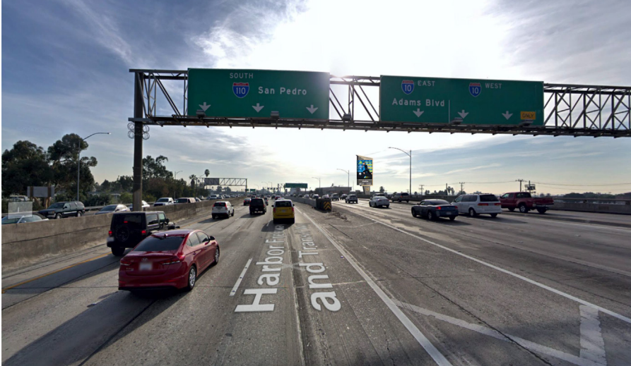
Photo C.320: I-110 Southbound view at 320 feet from 12th Place Sign
