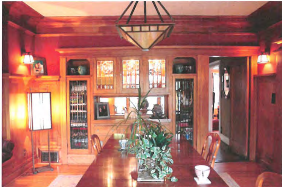
Dining room: North wall; east wall breakfront with art glass doors; beveled mirror & wood insets and drawers, double swing door to kitchen; south entry to dining room; deep ceiling molding; plate rail; hardwood floor, view east.
