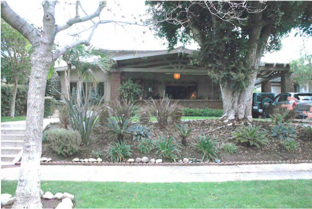
West elevation of 226 S. St. Andrews Place.
