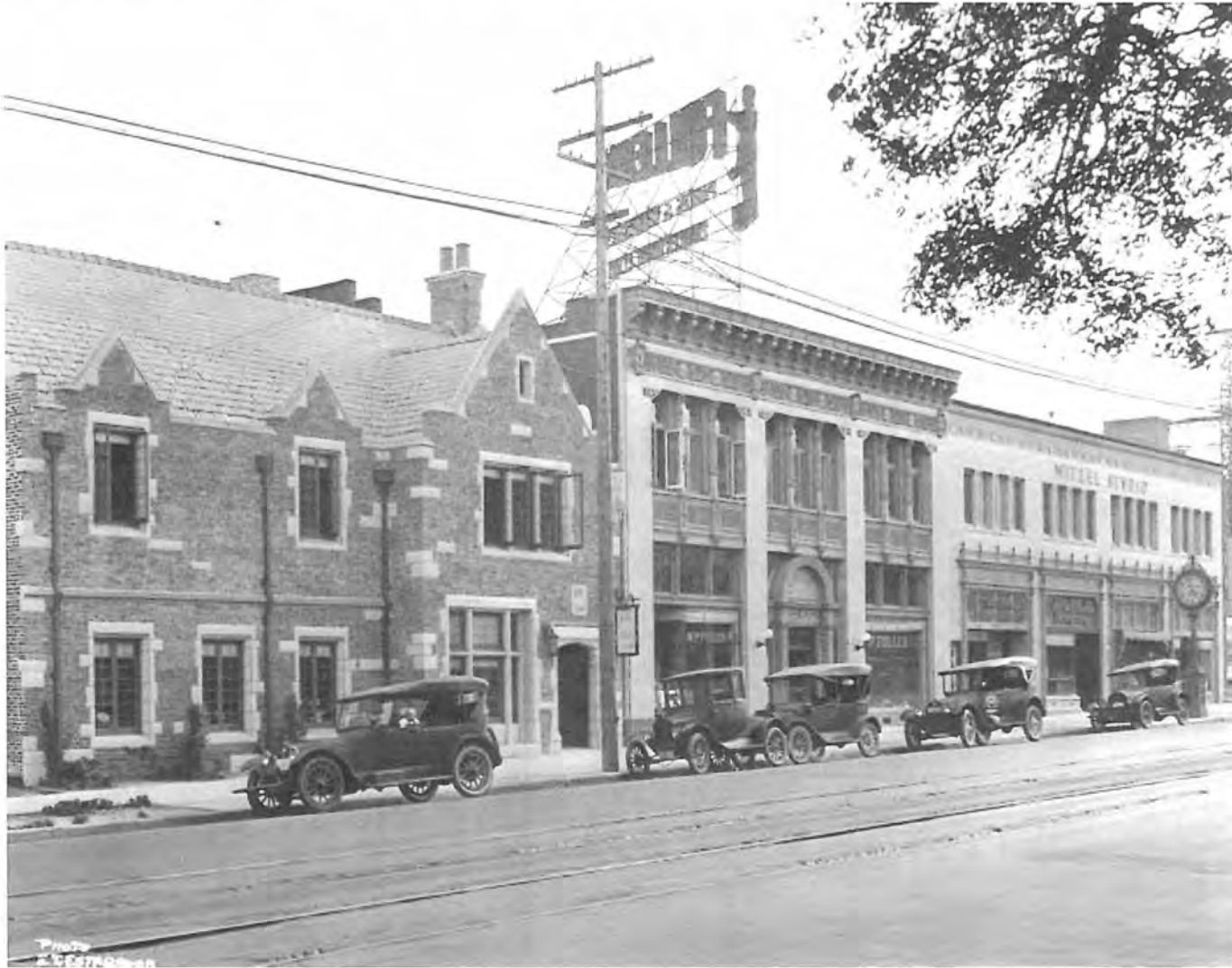
Witzel Studio, at left: 6324 Hollywood Boulevard, Hollywood, Los Angeles, CA, c. 1920s. [demolished]
