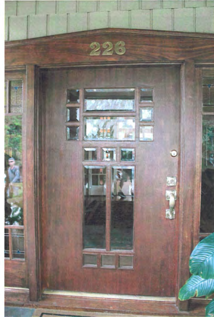
Entry door from west raised porch featuring multi-pane beveled glass; sidelights either side, view east.
