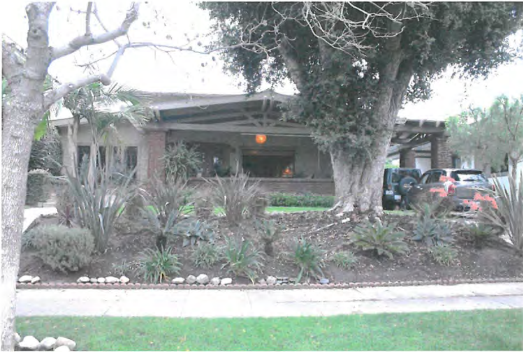
Front/west façade of residence across front lawn with second story portion peeking over north side of porch; porte-cochere at south, view east.
