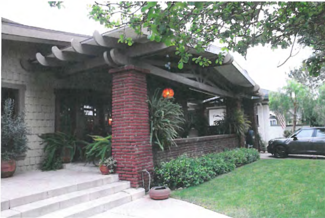
West, raised brick entry gabled porch in Oriental style with Oriental beam ends: steps down to lawn, view southeast.
