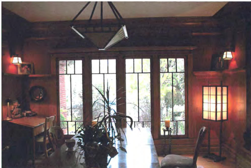
Dining room: South wall; west ribbon windows; deep ceiling molding; plate rail atop tall wainscoting; hardwood floors; northwest corner, view west.
