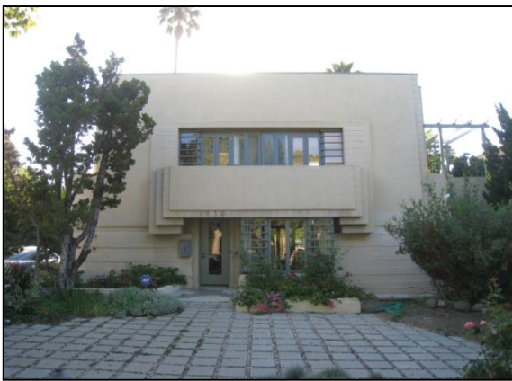
Primary, west elevation, view east
