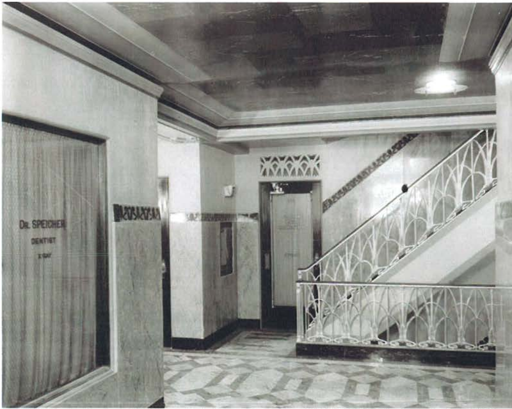
Wilshire Professional Building, historic upstairs lobby, 3875 Wilshire Boulevard, circa 1929
