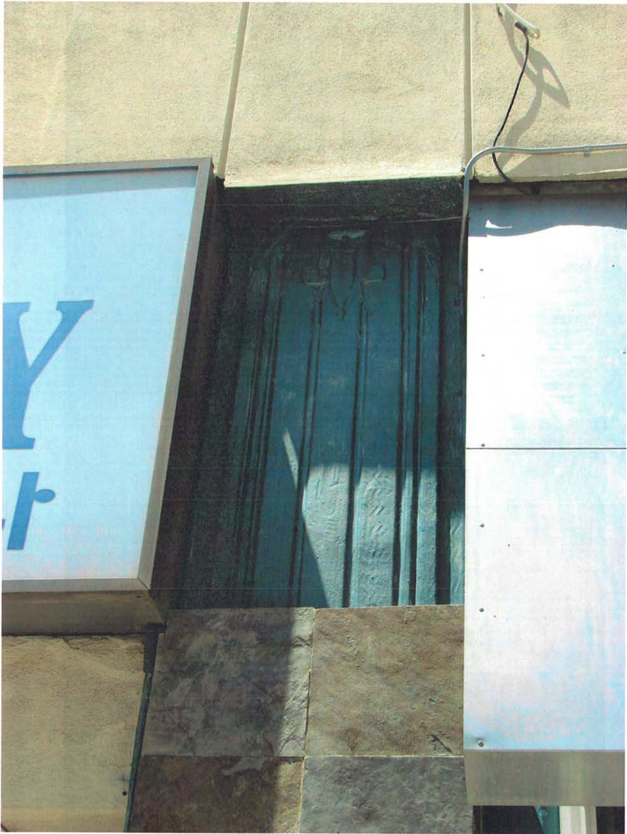
Wilshire Professional Building, original 1st floor facade hidden, 3875 Wilshire Boulevard, June 21, 2013
