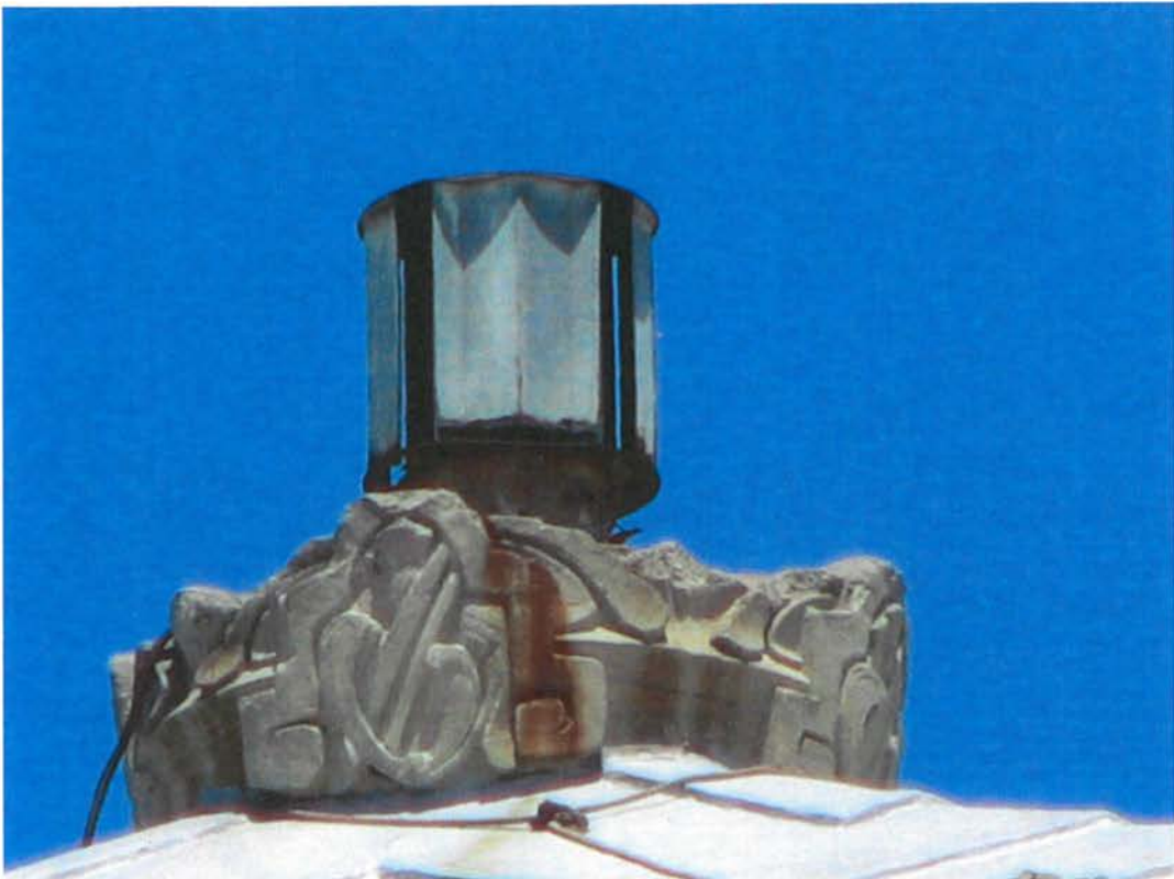
Wilshire Professional Building, rooftop light, 3875 Wilshire Boulevard, June 21, 2013
