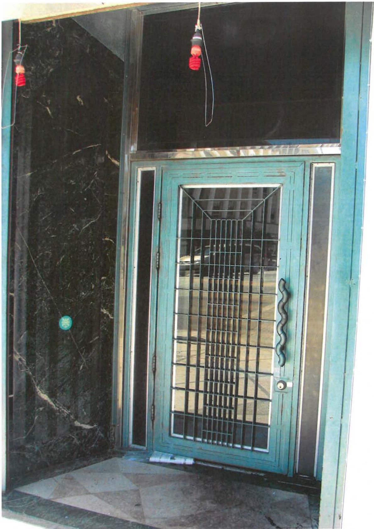
Wilshire Professional Building, current store entry, 3875 Wilshire Boulevard, June 21, 2013
