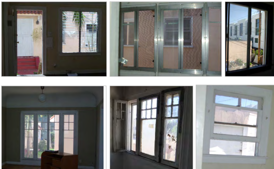
Figure 34 Altered windows and window frames (above); original window and frame types (below)
