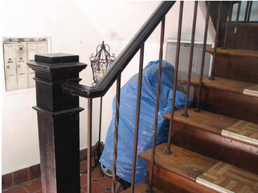
Norton Flats, entry foyer bannister, 412-420 N. Norton Avenue, August 27, 2015 (Photograph by Charles J. Fisher)
