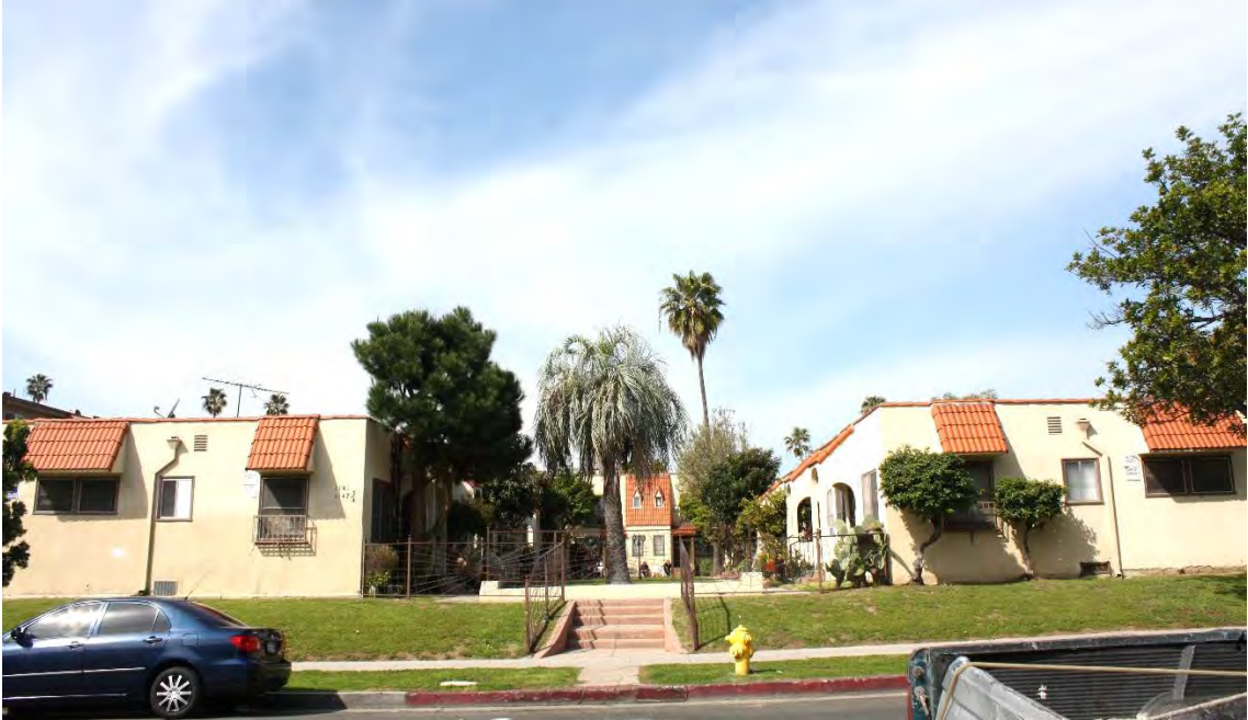
1141 - 1147 South Norton Avenue, 1923, J. C. De Witt, architect, protected by Country Club Park HPOZ.
