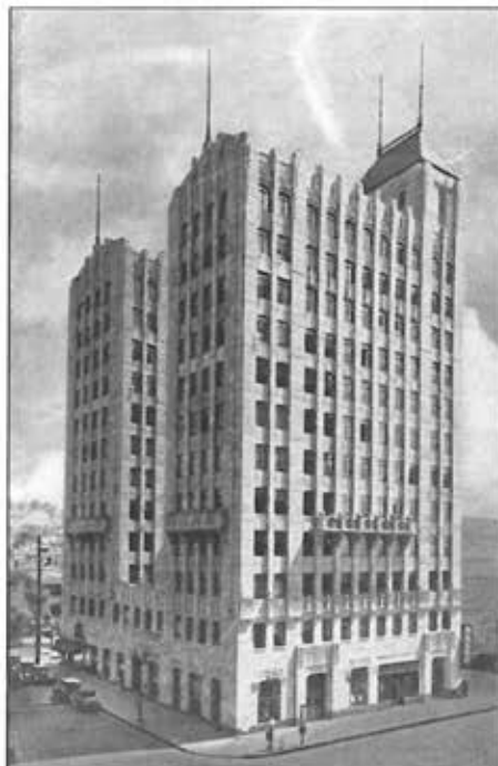
Image 6: 1930 rendering of south and west elevations, view northeast, note addition behind original tower to create U-shaped building (LAPL)
