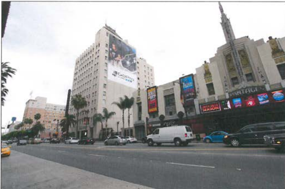
Photo 12: Bank of Hollywood / Equitable Building, south and east elevations, view northwest (Chattel 2014)
