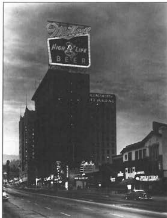
Image 14: c. 1930s photo of subject property with Vine Street development in foreground, view north (LAPL)
