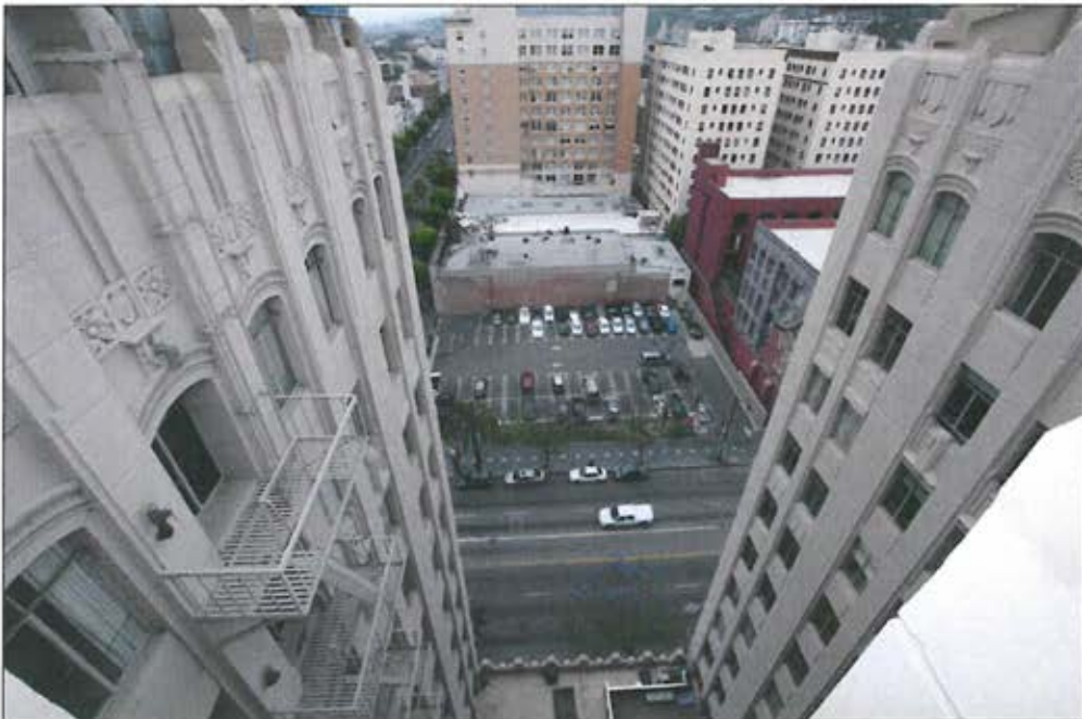
Photo 8: Bank of Hollywood / Equitable Building, west elevation, light court detail, view west (Chattel 2014)
