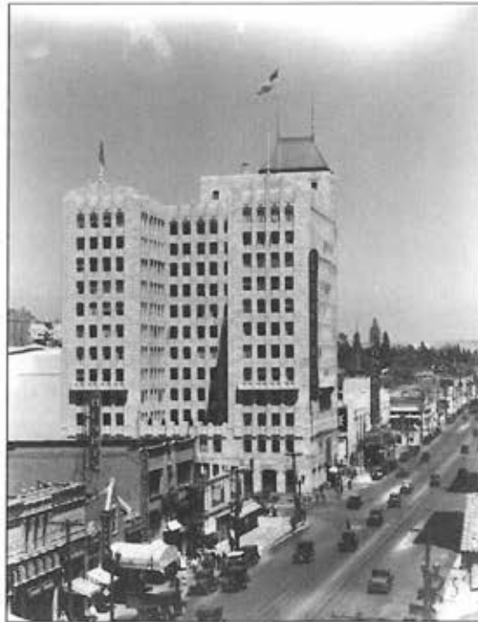
Image 9: c. 1931 photo of south and west elevations, view northeast (LAPL)
