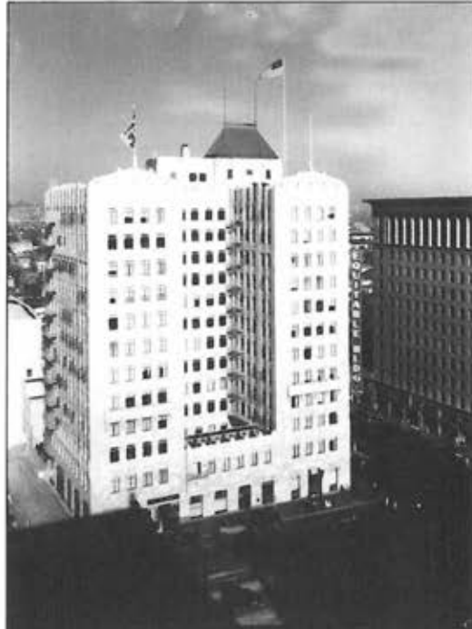
Image 10: c. 1931 photo of north and west elevations, view east (LAPL)
