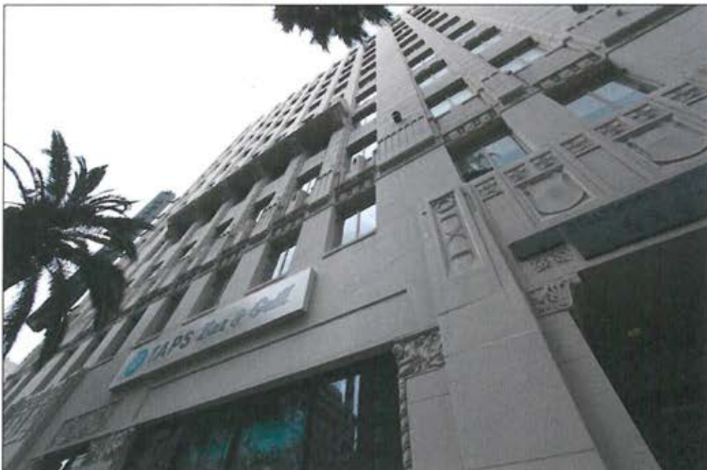
Photo 4: Bank of Hollywood / Equitable Building, south elevation, view north (Chattel 2014)
