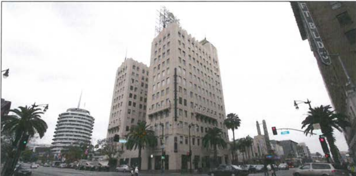
South and west elevations, view northeast (Chattel 2014)
