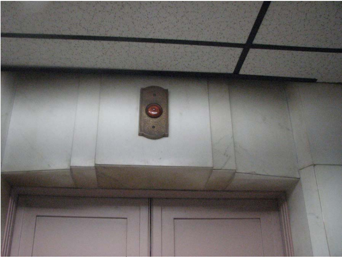
Sun Realty Company Building, elevator light 12 th floor, 629-33 S. Hill Street, June 2, 2009 (Photograph by Charles J. Fisher)
