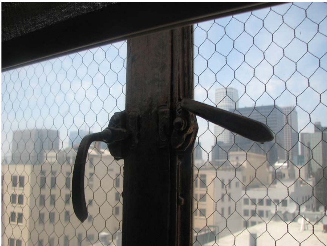
Sun Realty Co. Building hardware & glass in rear window, 629-33 S. Hill Street, June 2, 2009 (Photograph by Charles J. Fisher)
