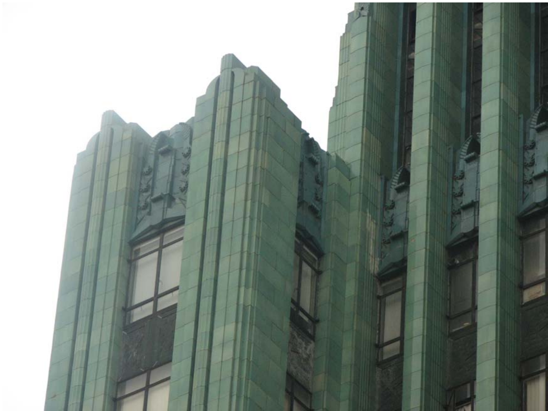
Sun Realty Company Building, 629-33 S. Hill Street, May 29, 2009 (Photograph by Charles J. Fisher)
