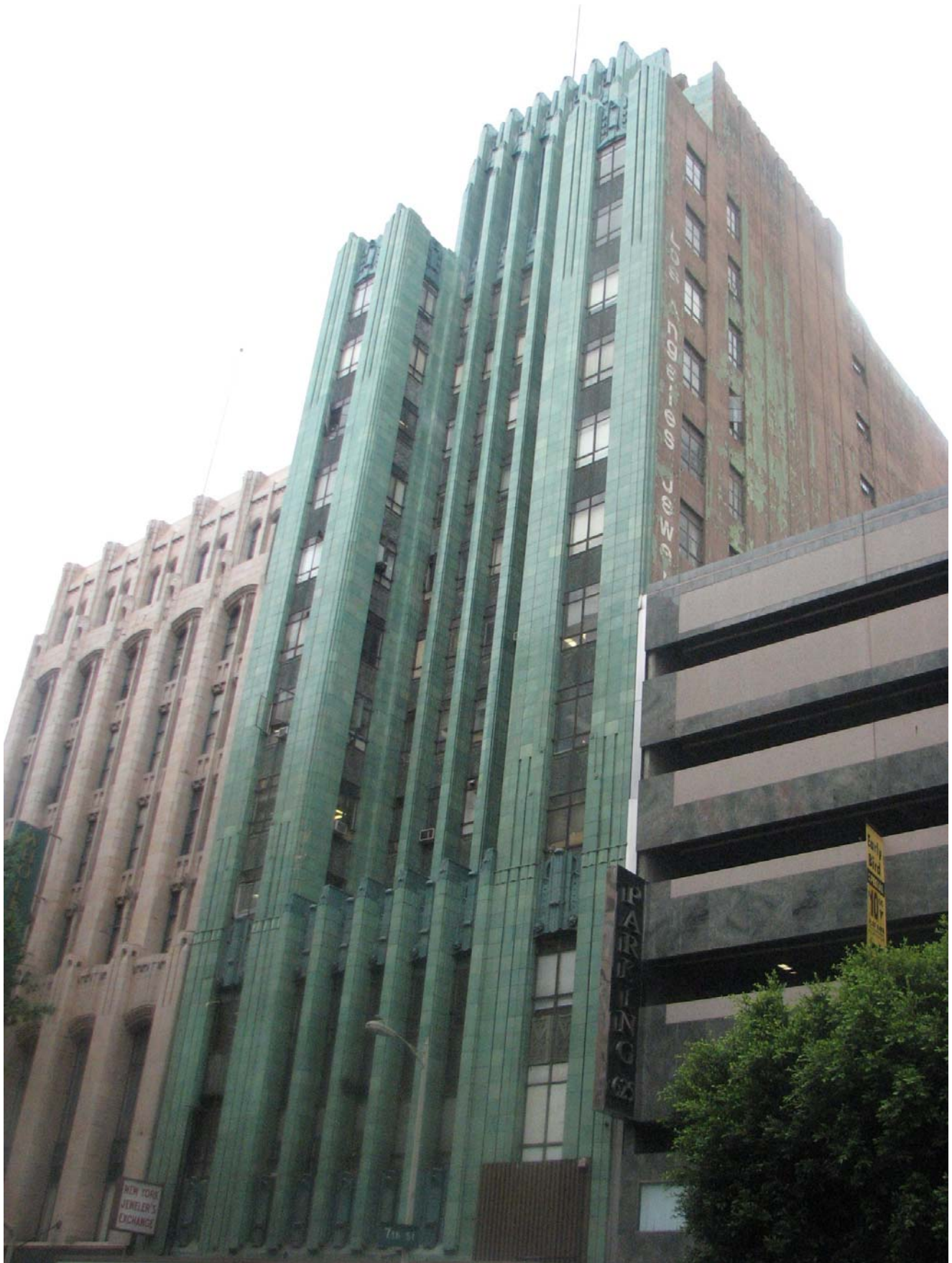
Sun Realty Company Building, 629-33 S. Hill Street, May 29, 2009 (Photograph by Charles J. Fisher)
