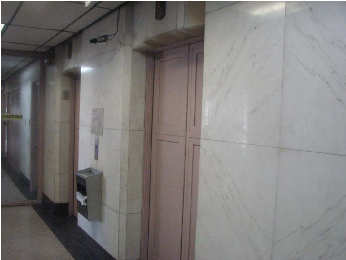
Sun Realty Company Building, 12 th floor elevator lobby, 629-33 S. Hill Street, June 2, 2009 (Photograph by Charles J. Fisher)
