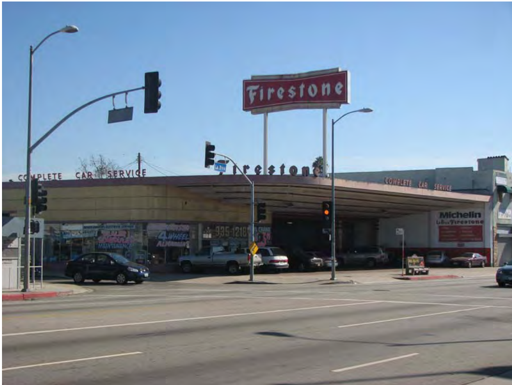
Firestone Tire Building, 800 S. La Brea Avenue, October 29, 2011 (Photograph by Charles J. Fisher)
