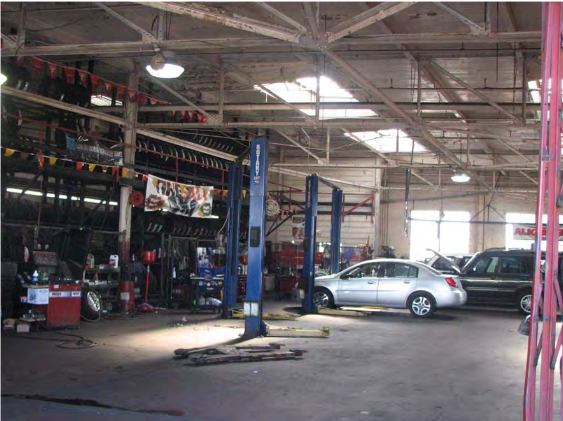
Firestone Tire Building, garage interior showing skylights, 800 S. La Brea Avenue, October 29, 2011 (Photograph by Charles J. Fisher)
