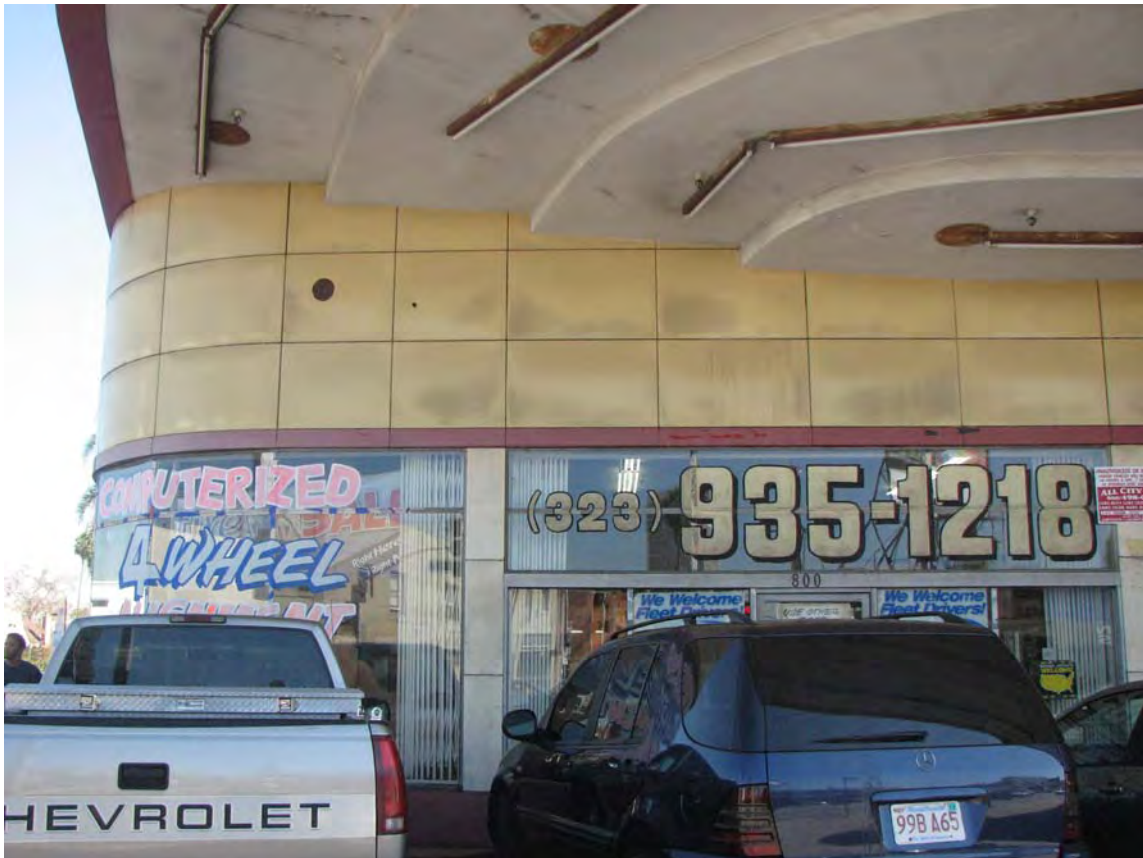
Firestone Tire Building, porcelain wall, 800 S. La Brea Avenue, October 29, 2011 (Photograph by Charles J. Fisher)
