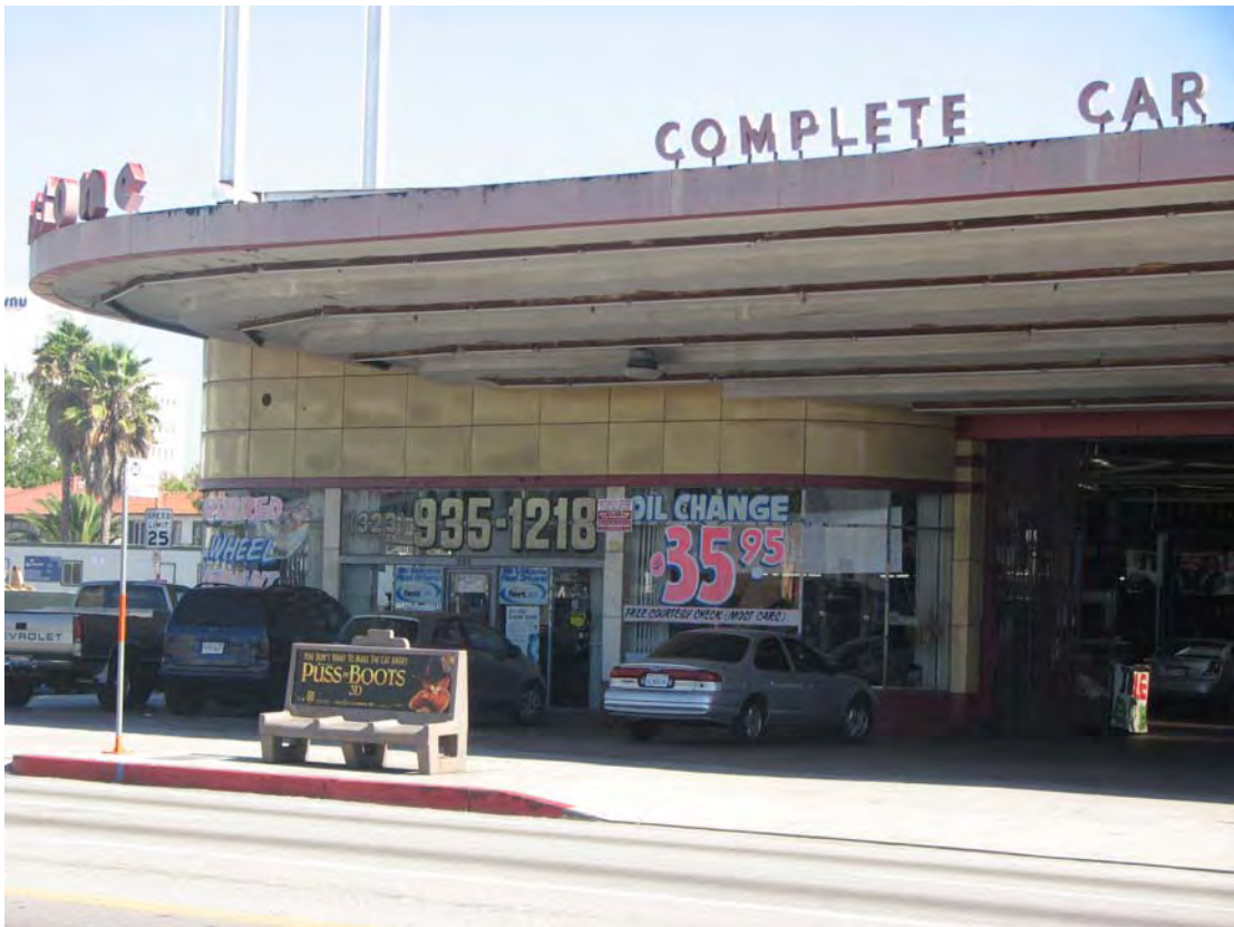
Firestone Tire Building, 800 S. La Brea Avenue, October 29, 2011 (Photograph by Charles J. Fisher)
