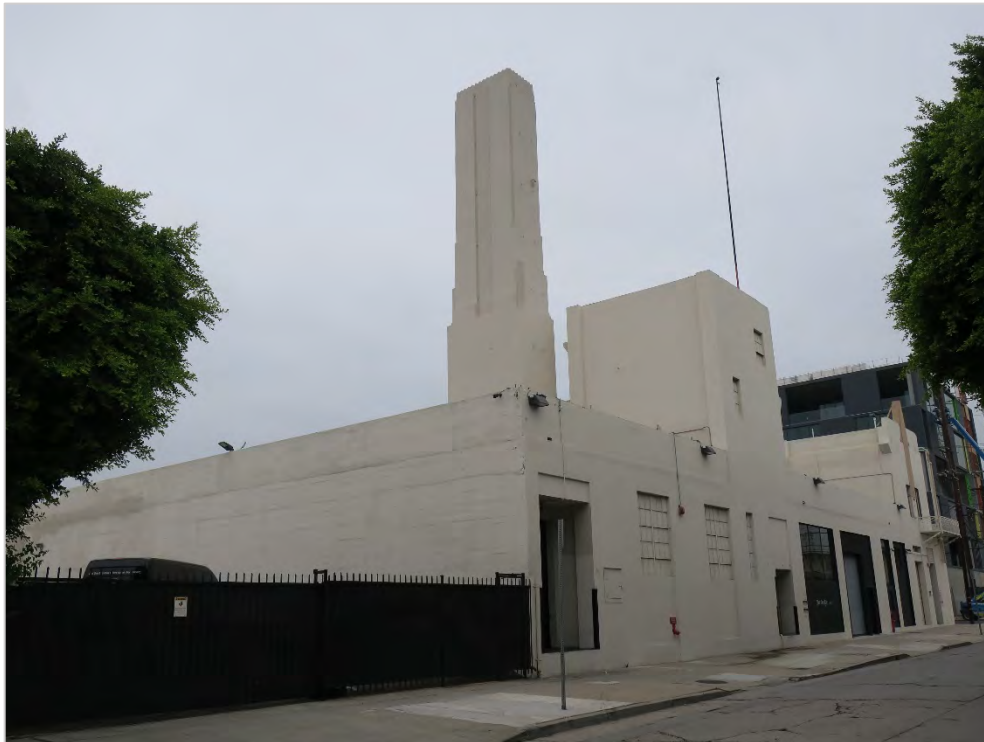
East façade and portion of south façade, view northwest (ARG, 2017).
