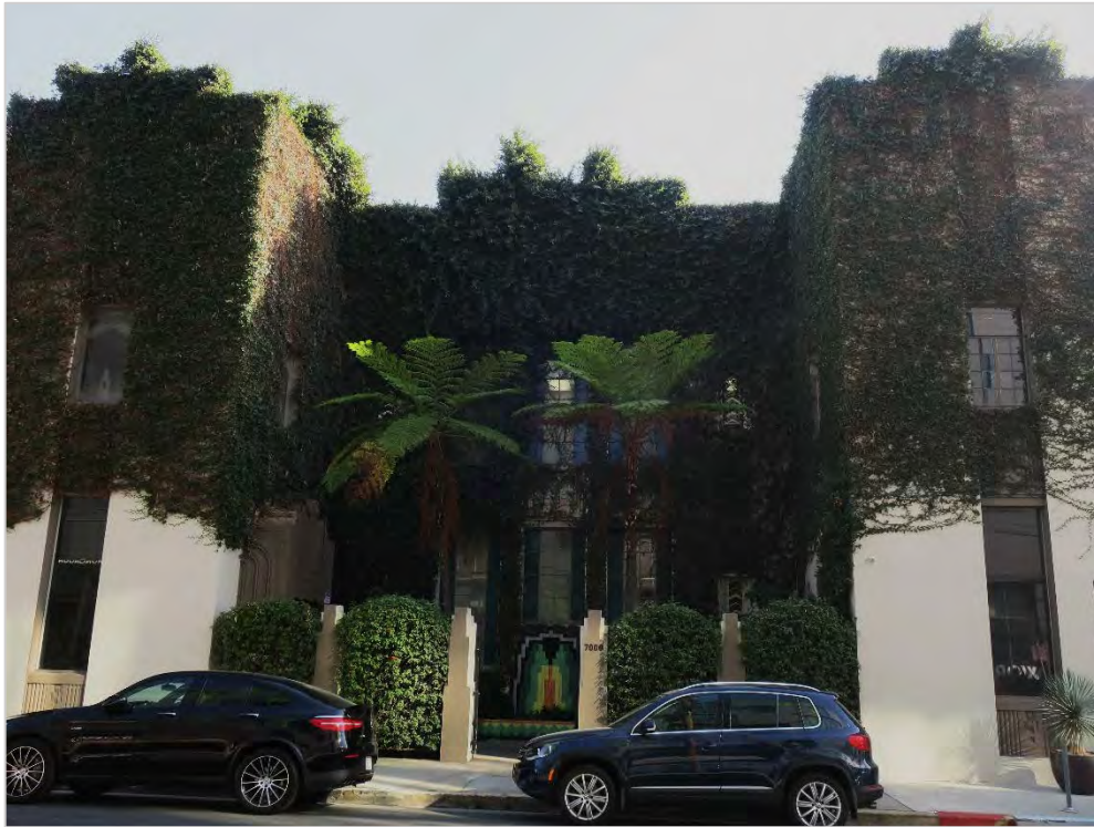
Primary (north) façade, central recessed courtyard entry, view south (ARG, 2019).
