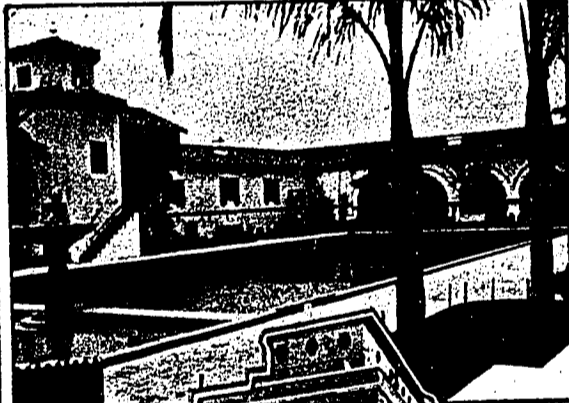
Bath House and Swimming Pool, Hotel Agua Caliente, Old Mexico, Wynn D. McAllister, Architect.
