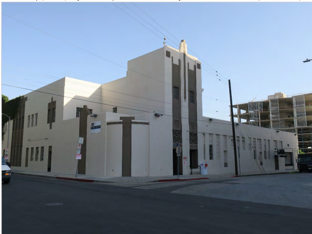
West façade and portion of north façade, view southeast (ARG, 2019).
