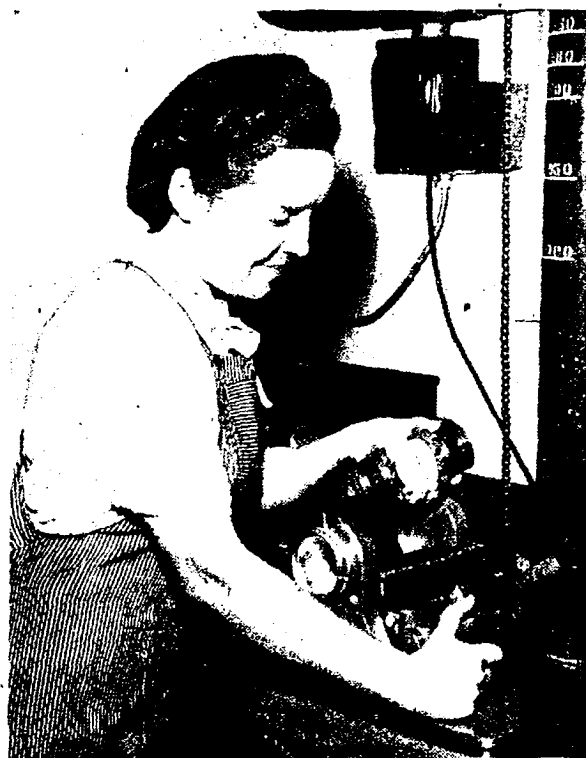
FAST WORK —Miss Lucille Rhodes makes load test on electric booster. It pushes or pulls shell belts through the chute at a speed of 840 rounds each minute.
