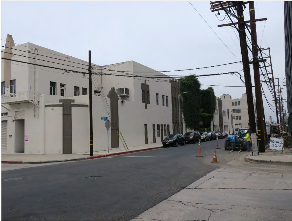
Primary (north) façade and portion of east façade, view southwest (ARG, 2017).
