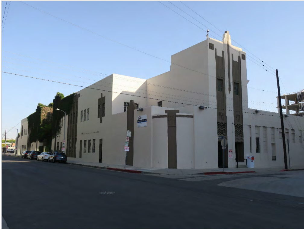
Primary (north) façade and portion of west façade, view southeast (ARG, 2019).
