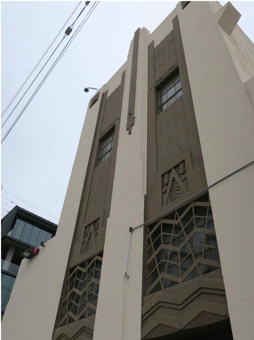
Art Deco details at west façade (ARG, 2017).
