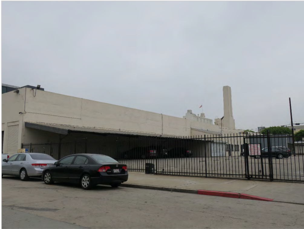
South façade, view northeast (ARG, 2017).
