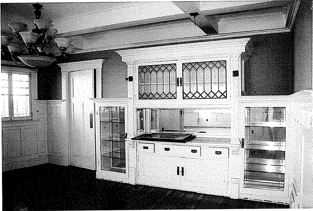
Dining room: North, east and south walls, viewed to east.
