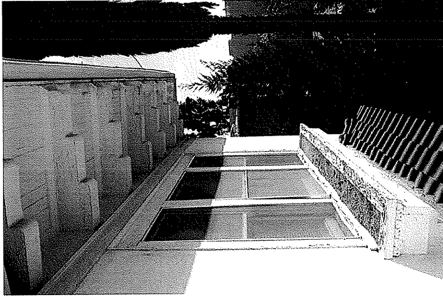
View to south from second level veranda, with projecting eaves w/ tri-step beam ends, window box with egg & dart border, and brackets beneath, and tiled mini roof above downstairs windows.
