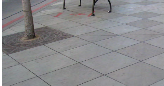
Example of Scored Integral Colored Concrete
