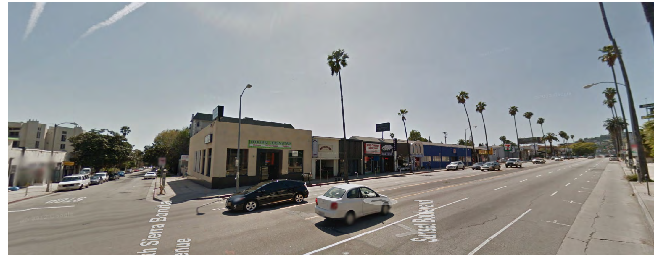
SITE PHOTO G 1" = 1'-0"
