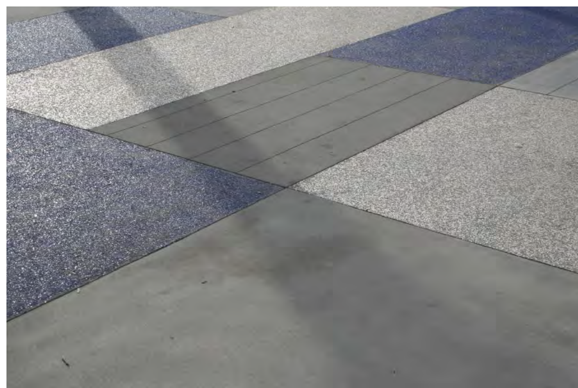
A Concrete paving with two colors & textures
