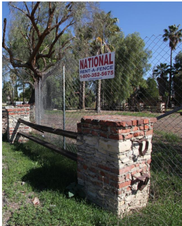
Figure 7: Detail of the historic stone and brick pilasters with wood split rail fence associated with the Canoga Mission Gallery, 2016 (Chattel, Inc.)
