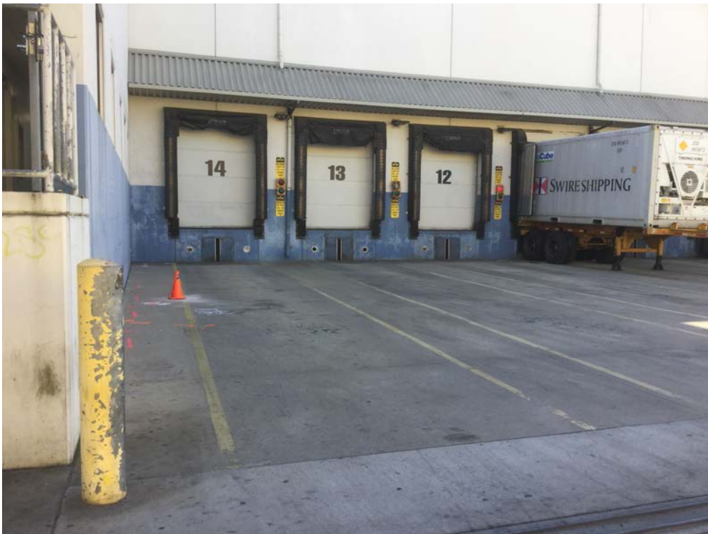
Loading dock along Industrial Street; view to the south. 1562 Industrial Street, Los Angeles, CA 90021
