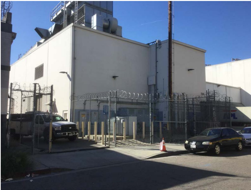
Eastern portion of subject building; view to the southwest. 1570 Industrial Street, Los Angeles, CA 90021
