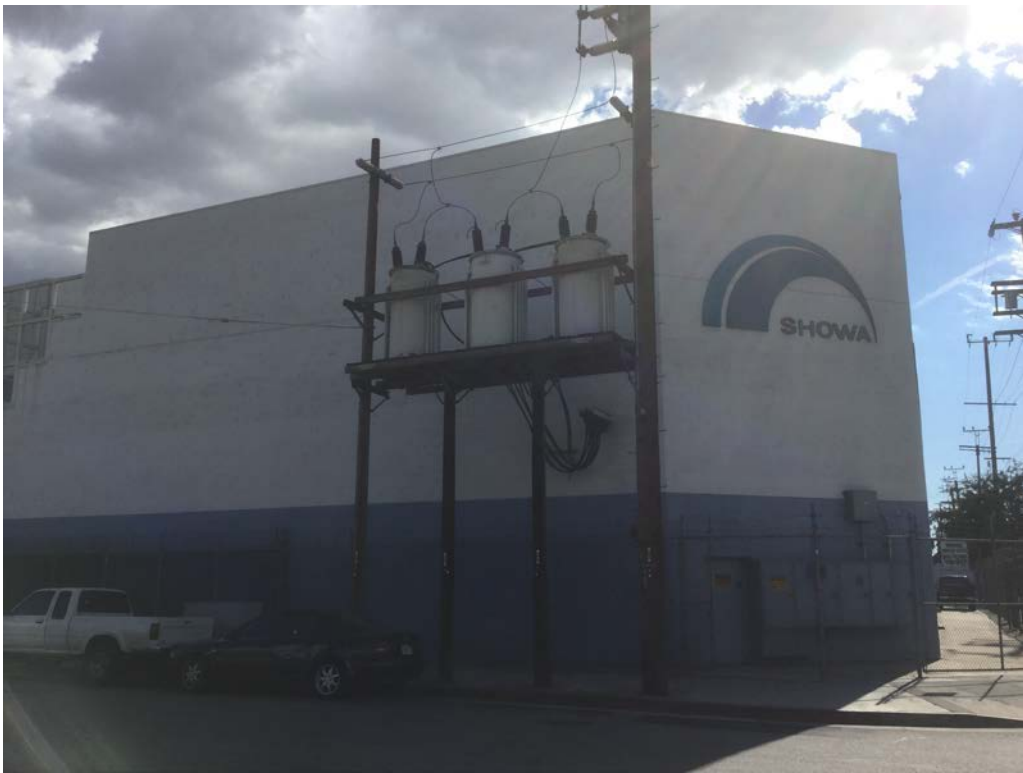
Subject building from Industrial Street; view to the southwest. 668 Alameda Street, Los Angeles, CA 90021
