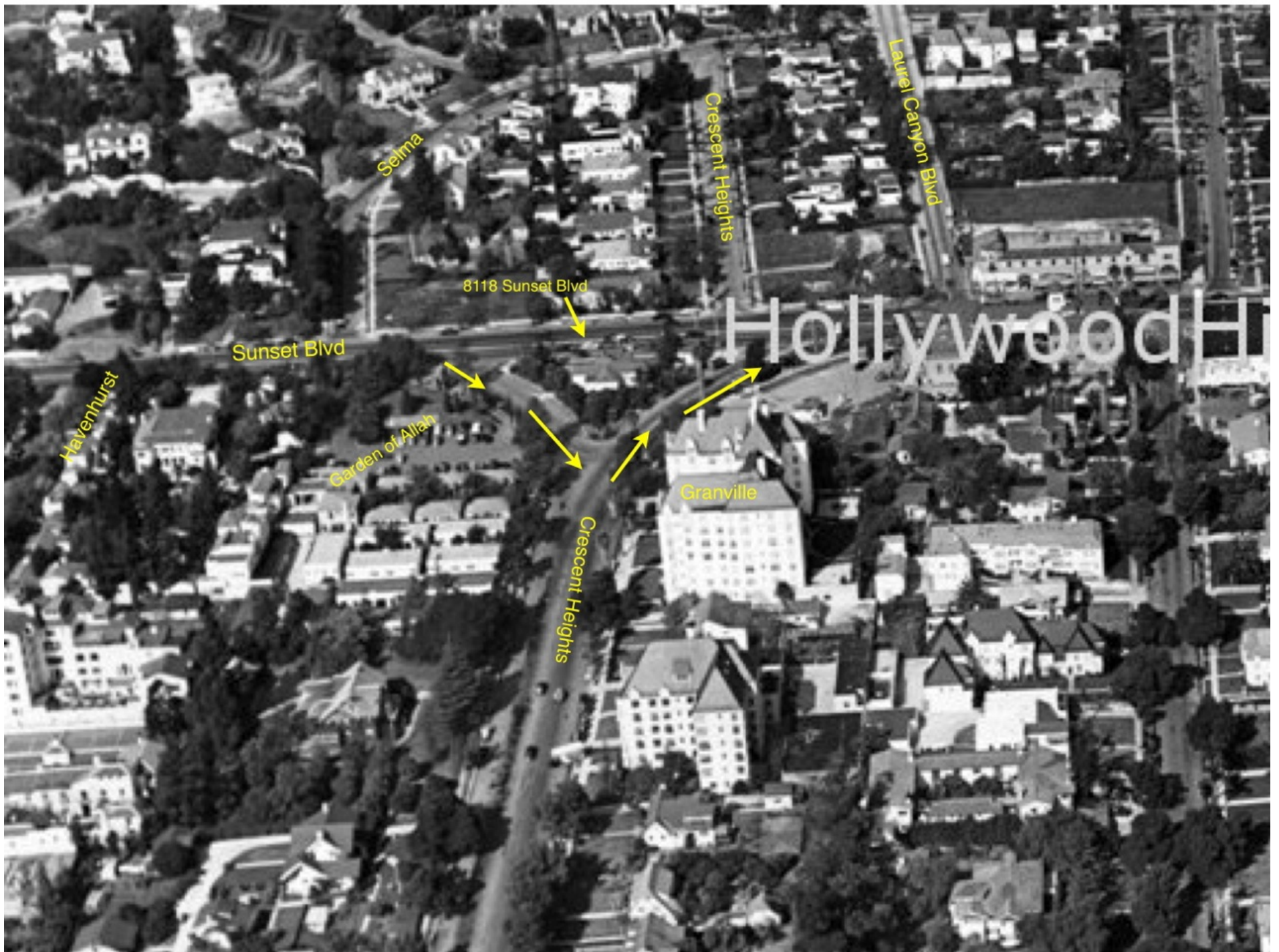
Year 1941 Crescent Heights and Sunset Blvd, 8118 Sunset Blvd
