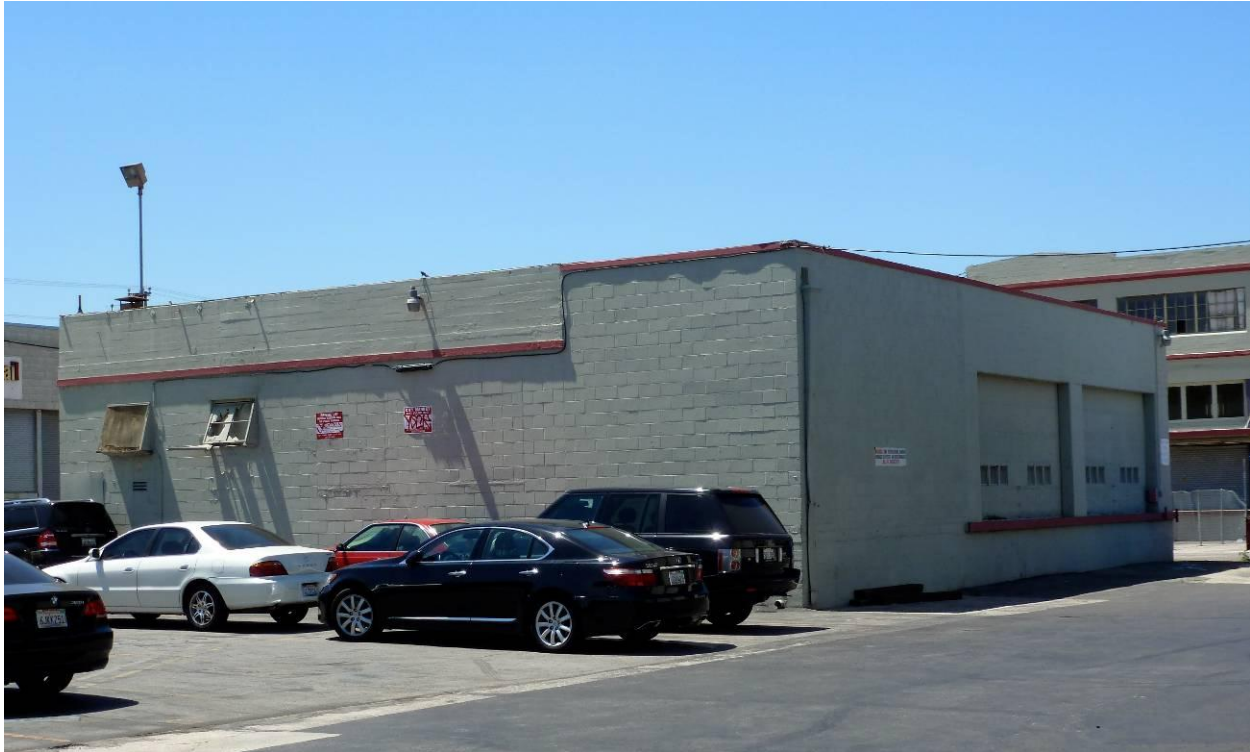
Figure 9: Building 4B, northeast and northwest elevations. Source: GPA.
