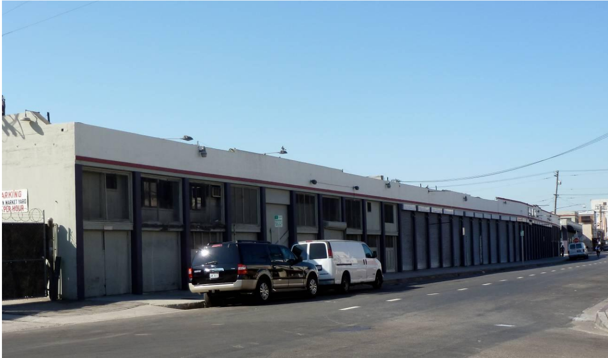
Figure 7: Building 3, 1040-1076 San Julian Street, northwest elevation. Source: GPA.
