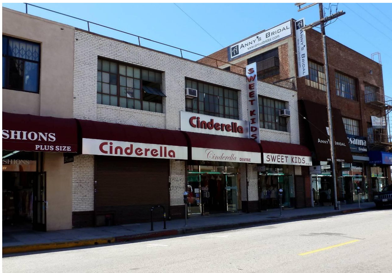
Figure 11: Building 6, 1142 San Julian Street, northwest elevation. Source: GPA.
