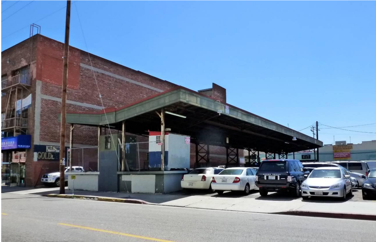
Figure 13: Structure 8, 1150 San Julian Street, northwest and southwest elevations. Source: GPA.
