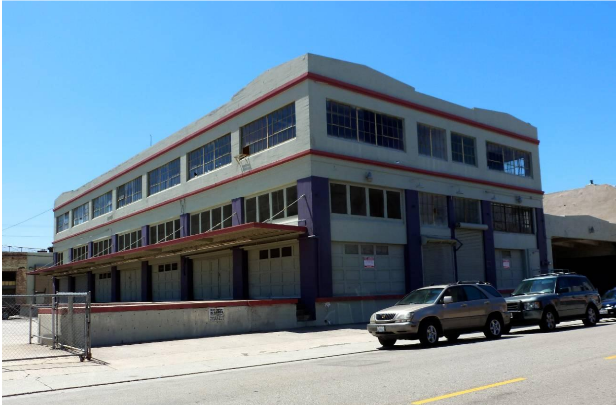
Figure 10: Building 5, 1122 San Julian Street, northwest and northeast elevations. Source: GPA.
