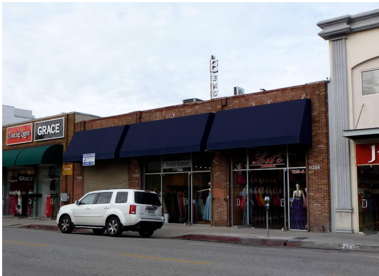
Figure 6: Building 2, 1125 San Julian Street, southeast elevation. Source: GPA.
