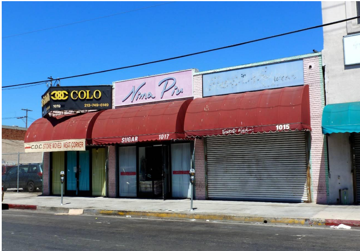
Figure 5: Building 1, 1015 San Julian Street, southeast elevation. Source: GPA.
