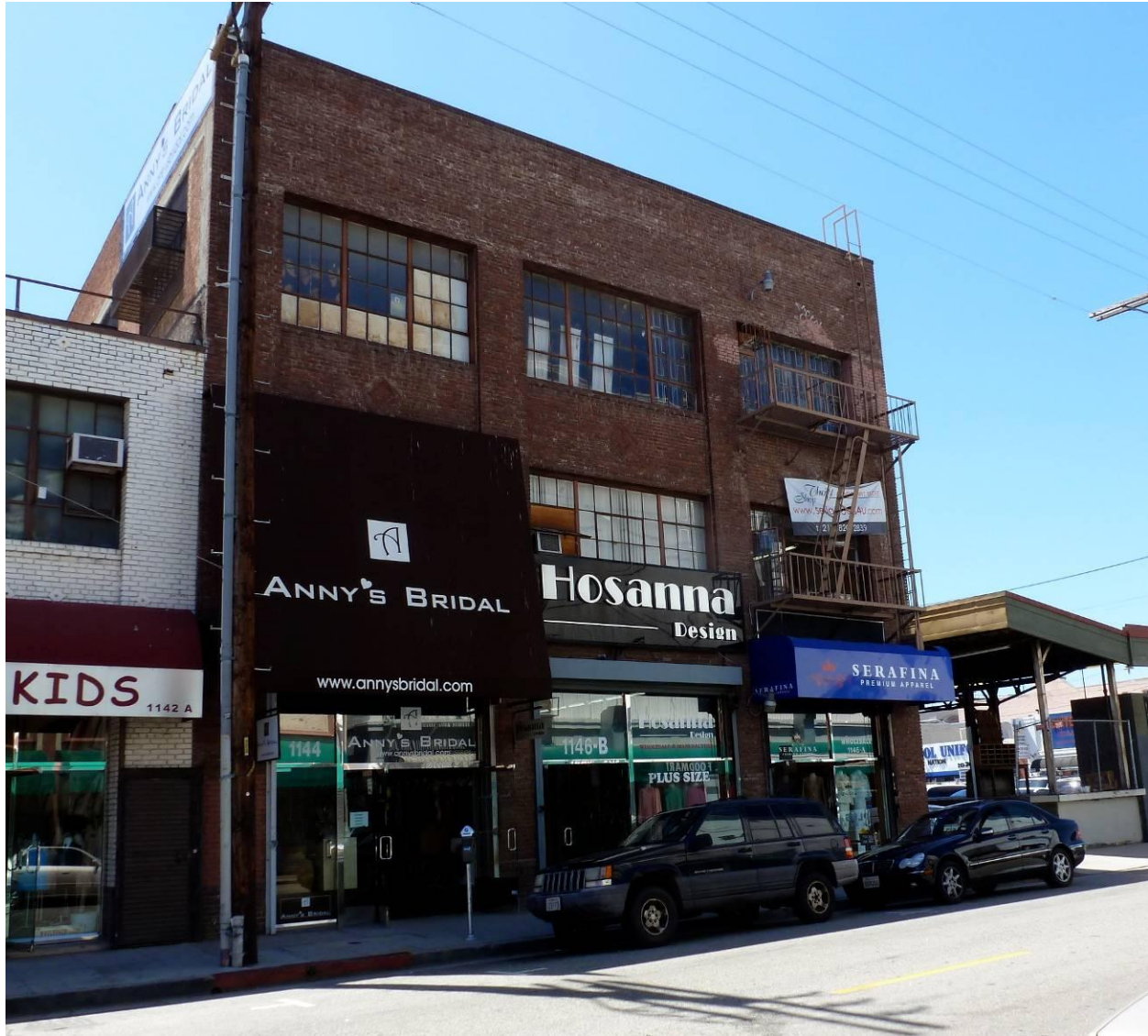
Figure 12: Building 7, 1146 San Julian Street, northwest elevation. Source: GPA.
