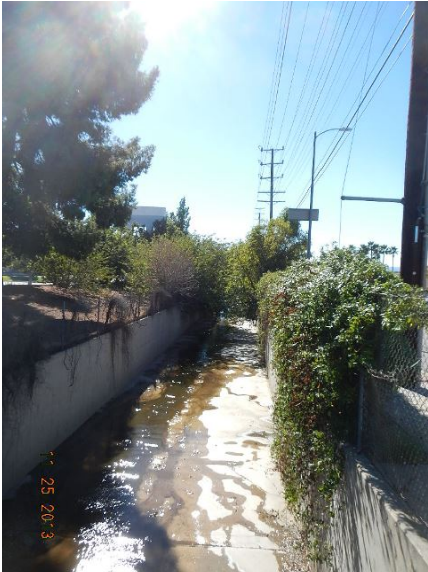
Looking south down the flood control channel.
