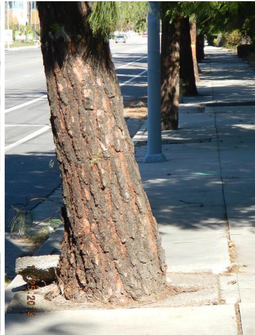
The collars around the base are girdling the trunks.
