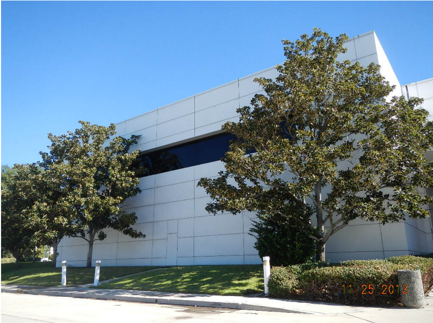
Magnolias along the west side of the building are adequately healthy.
