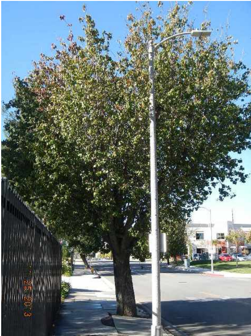
Note the lifted sidewalk.
