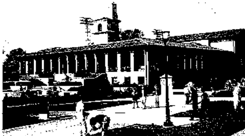
Figure 6. Johnson Student Center/Freeman College Union, Facing northwest
