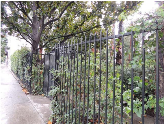
Montecito Apartments, 6650 Franklin Avenue Fence of landscaped garden area looking southeast from Franklin Avenue,
