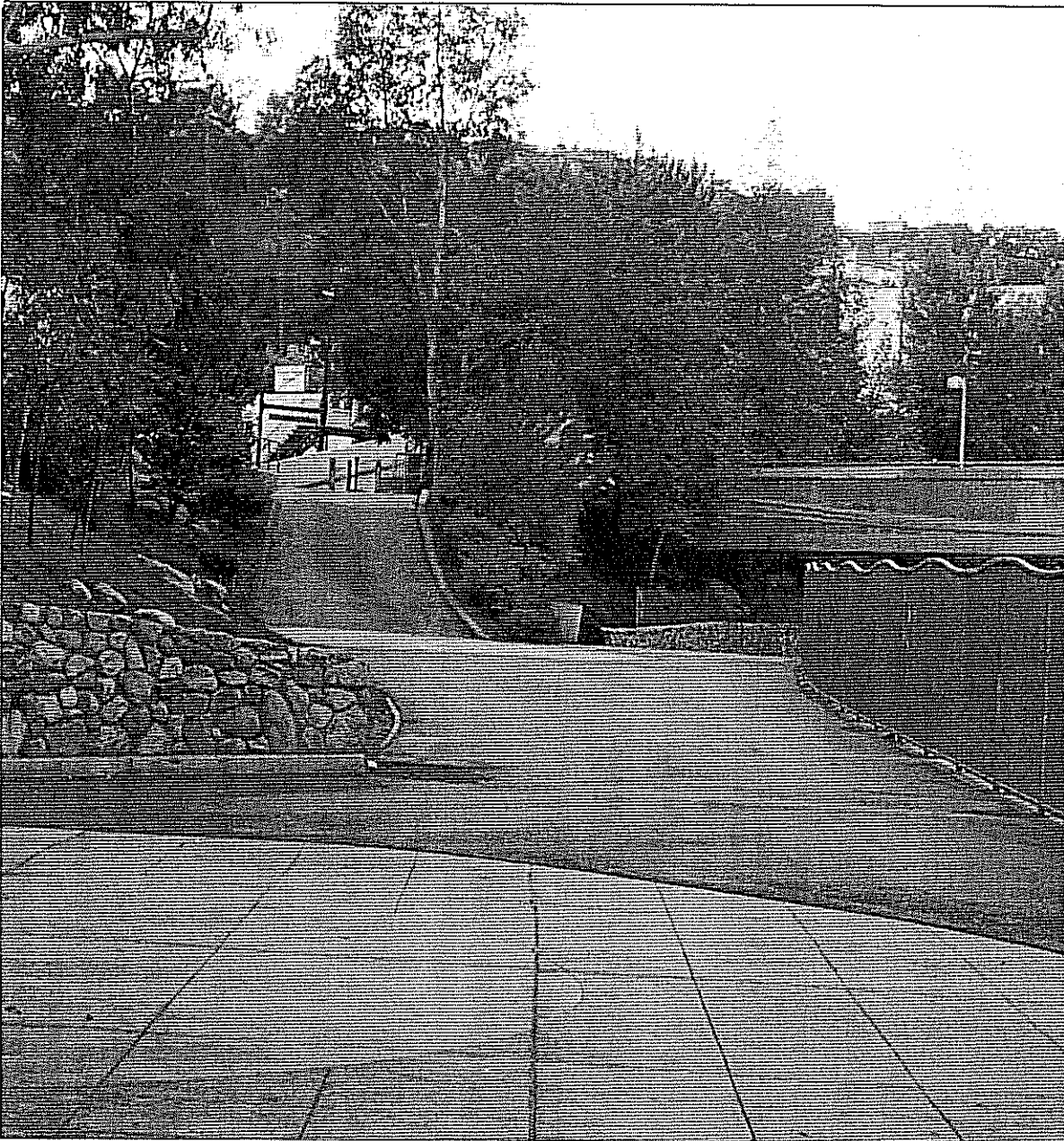
VIEW TOWARDS EXISTING PEDESTRIAN BRIDGE WEST OF PARKING STRUCTURE
