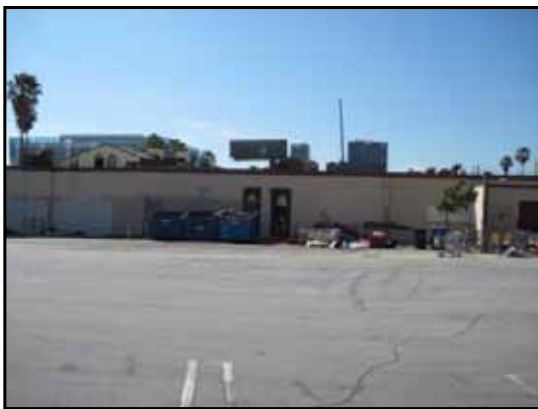
51 : Adjacent property to north of parking lot A - Vacant restaurant
