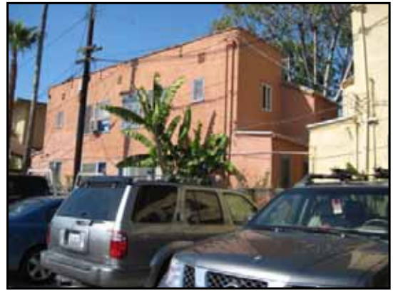
50 : Adjacent property to north of parking lot A - Residential
