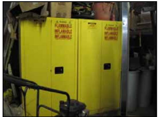
30 : Flammable storage in maintenance area under building
