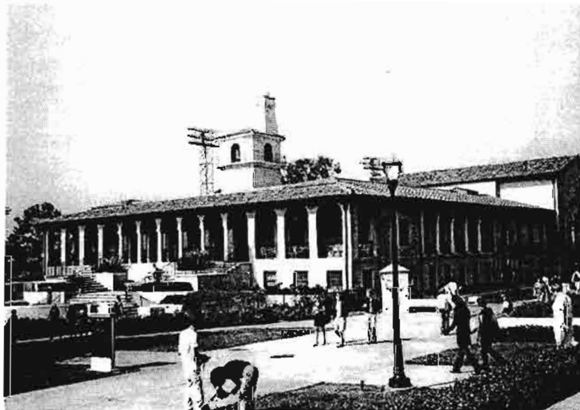
Figure 6. Johnson Student Center/Freeman College Union, facing northwest
