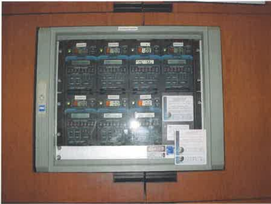
17. Methane detection system inside the Whole Foods Store.
