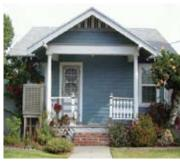
The central door opening has been filled-in & a new door has been placed off-center.
