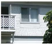
The siding added to the bottom of the window does not match the original shingle siding.
