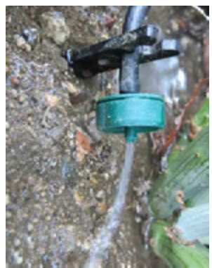
DRIP TUBING WITH 1 OR 2 DRIP EMITTERS) PER SHRUB
