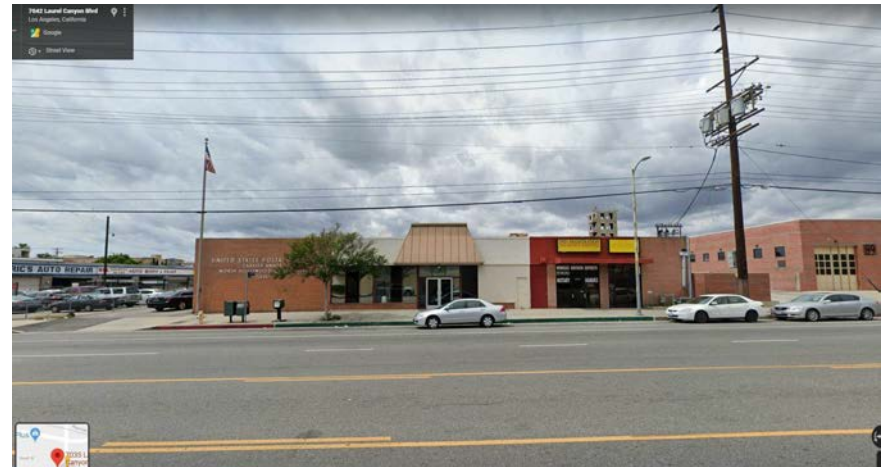
VIEW 2 - ON LAUREL CANYON BLVD TOWARDS SITE
