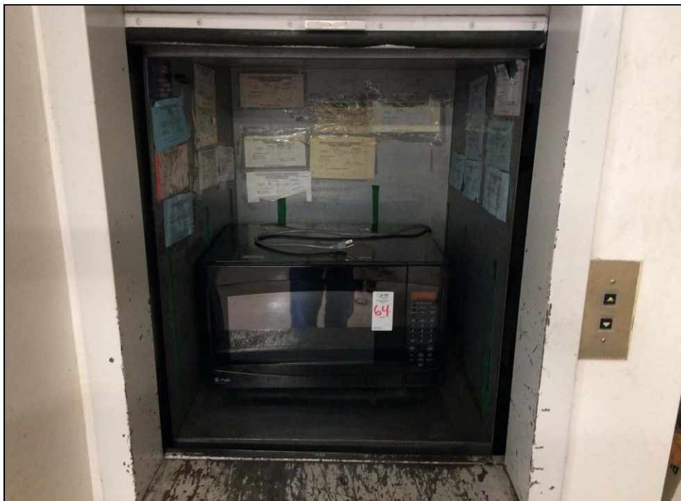
Photo 16: View of dumbwaiter within the two-story building.
