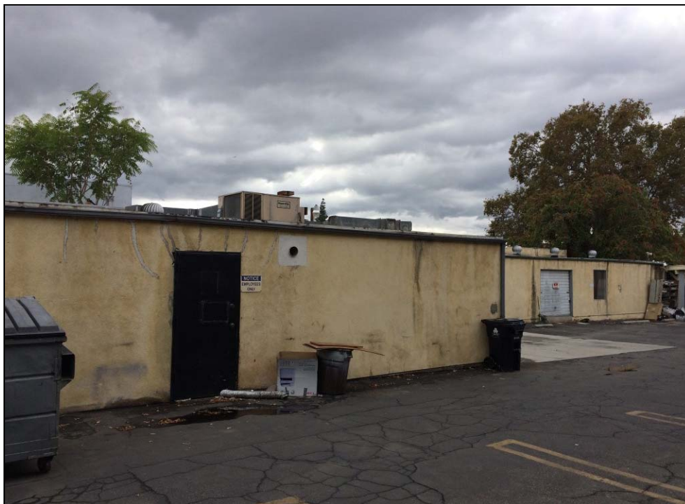
Photo 6: View of single-story storage buildings.
