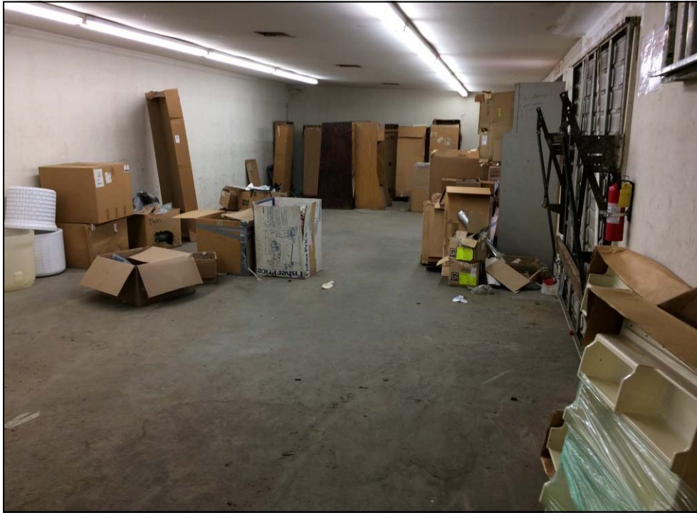
Photo 19: View of interior portion of the single-story storage building.
