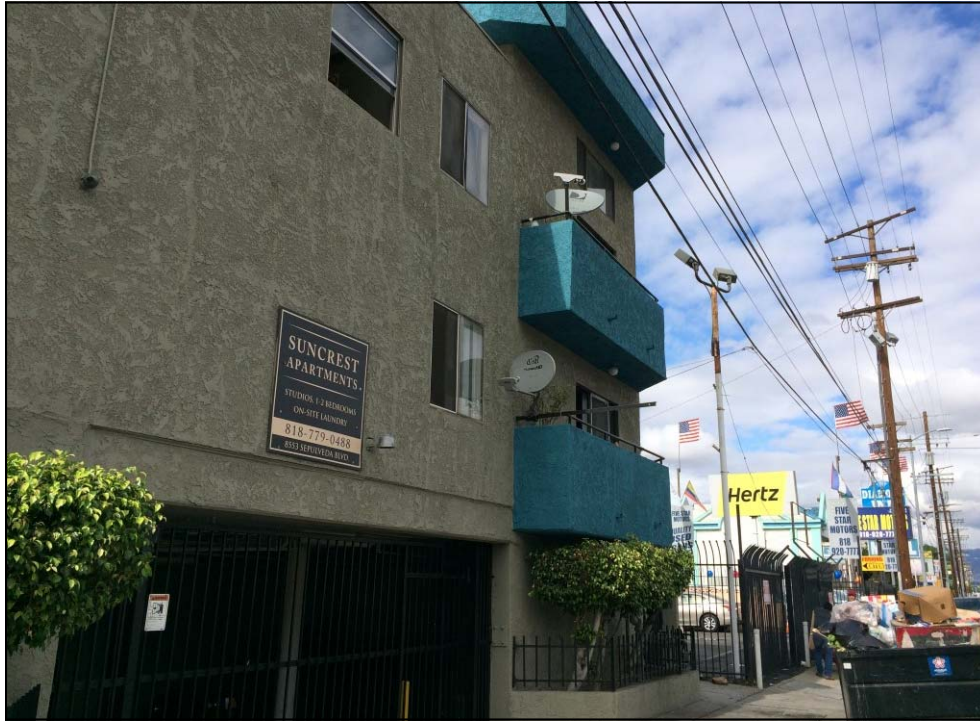
Photo 25: View of the adjacent property to the north.
