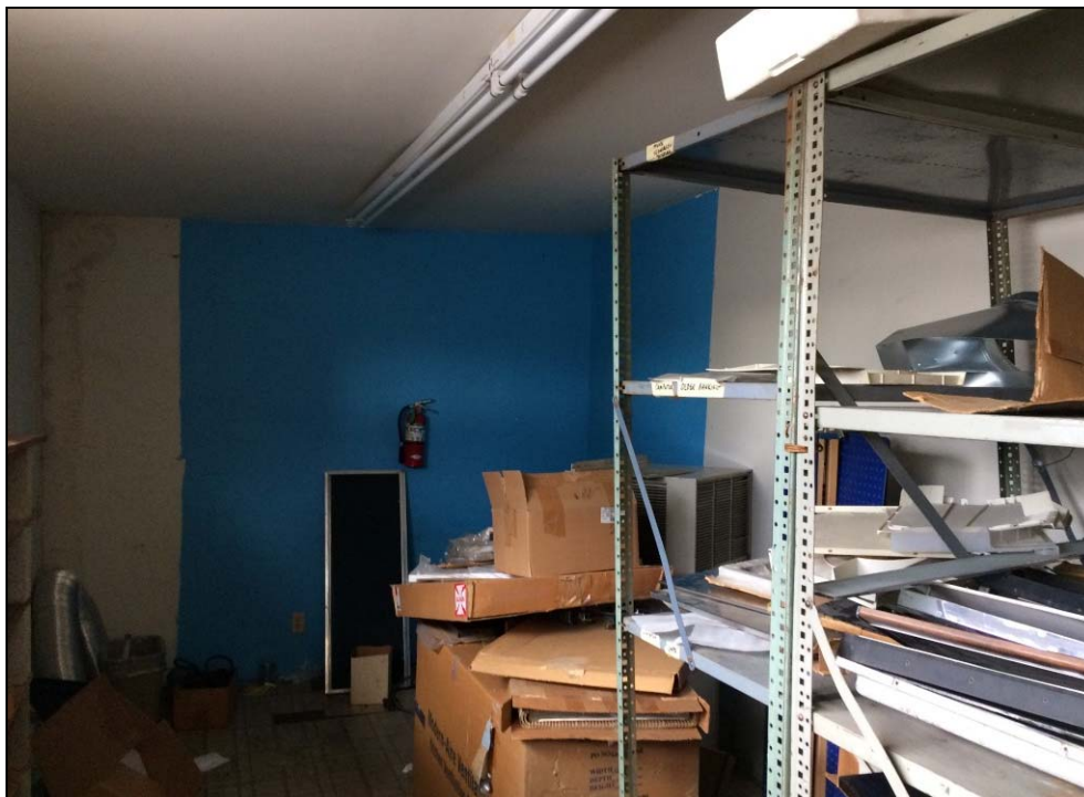
Photo 14: View of interior portion of the two-story building.
