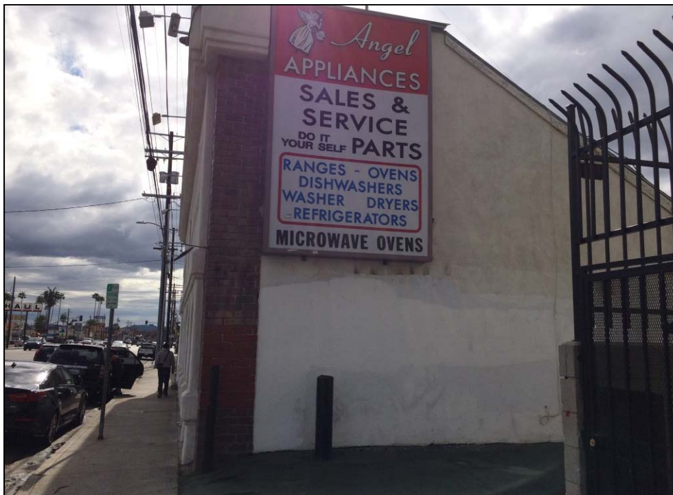
Photo 2: View of the eastern portion of the subject property looking south.
