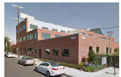
Figure 5 Industrial building on Califa Street.. Source: DCP
