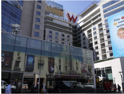
The W Hotel is located in the Regional Center and the Hollywood Signage Supplemental Use District
