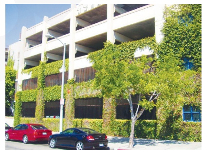
Screening above ground parking lots with greenery makes for a more pleasant walking experience
