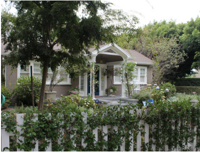
Sunset Square includes a variety of historic architectural styles, like this example of colonial revival
