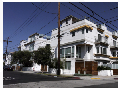
New multi-family residential housing units in Hollywood
