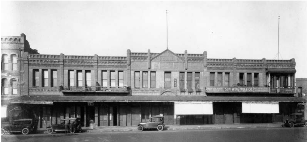
Garnier Building, n.d. Los Angeles Public Library, Security Pacific National Bank Collection.
