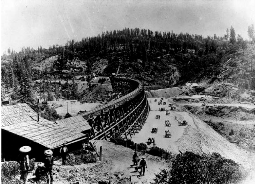
Chinese workers constructing a railroad bridge, n.d. (Los Angeles Public Library, Security Pacific National Bank Collection).
