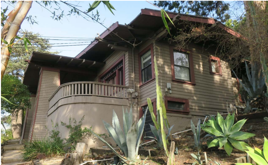
Pleasance House, view northeast of the primary façade, porch, and south façade (ARG, 2019).
