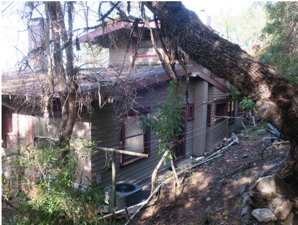
Pleasance House, view northwest of the east façade (ARG, 2019).
