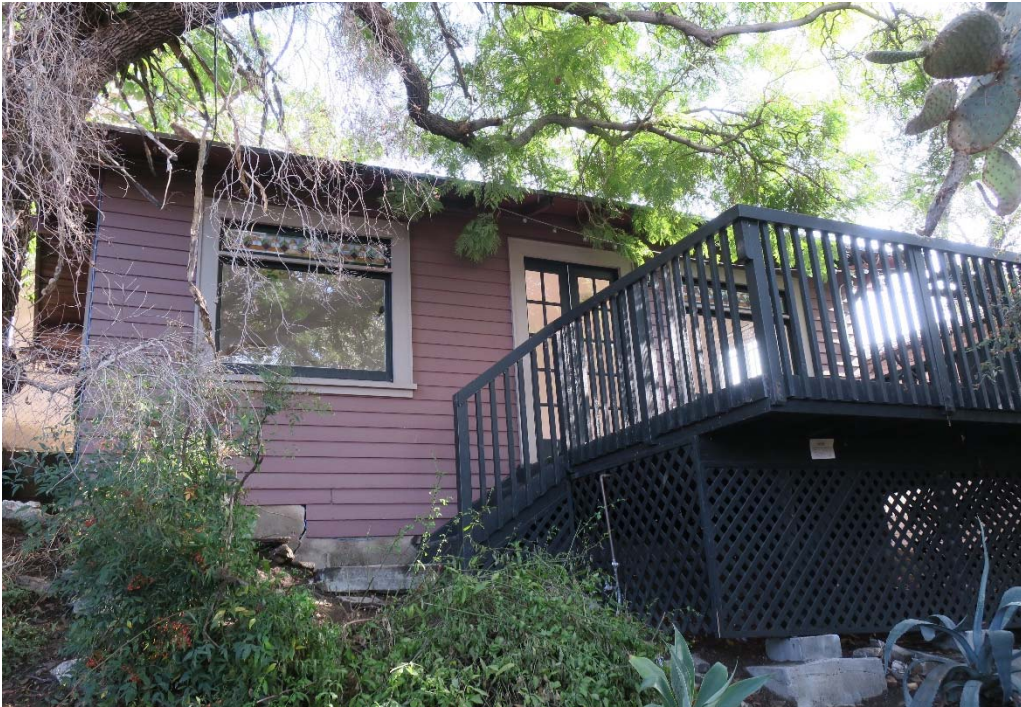
Pleasance House guesthouse, view southeast of the west (primary) façade (ARG, 2019).
