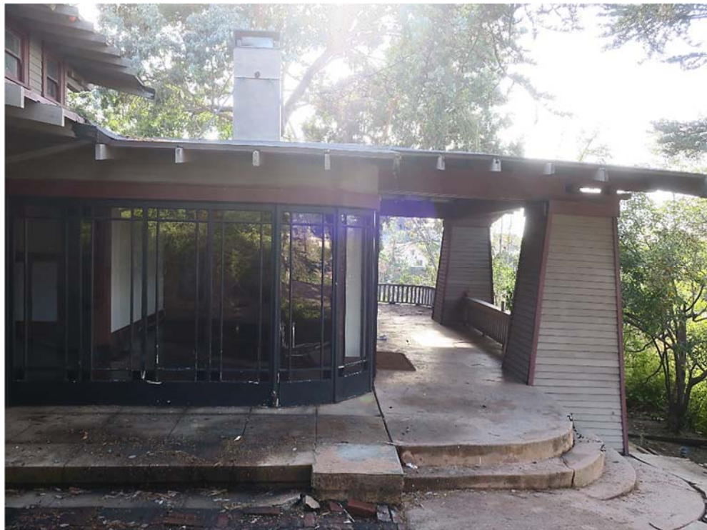
Pleasance House, view south of the front porch and group of canted fixed windows (ARG, 2019).
