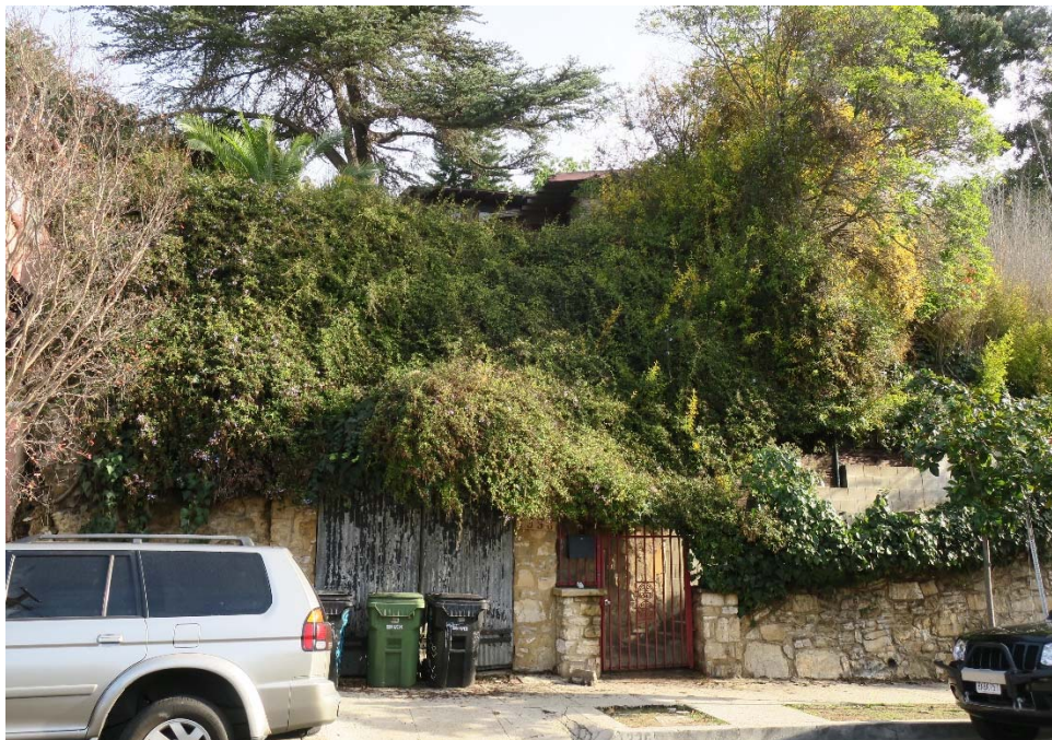
Pleasance House, view east from street level. Note the original built-in garage with non-original doors (left) and stone retaining wall (ARG, 2019).
